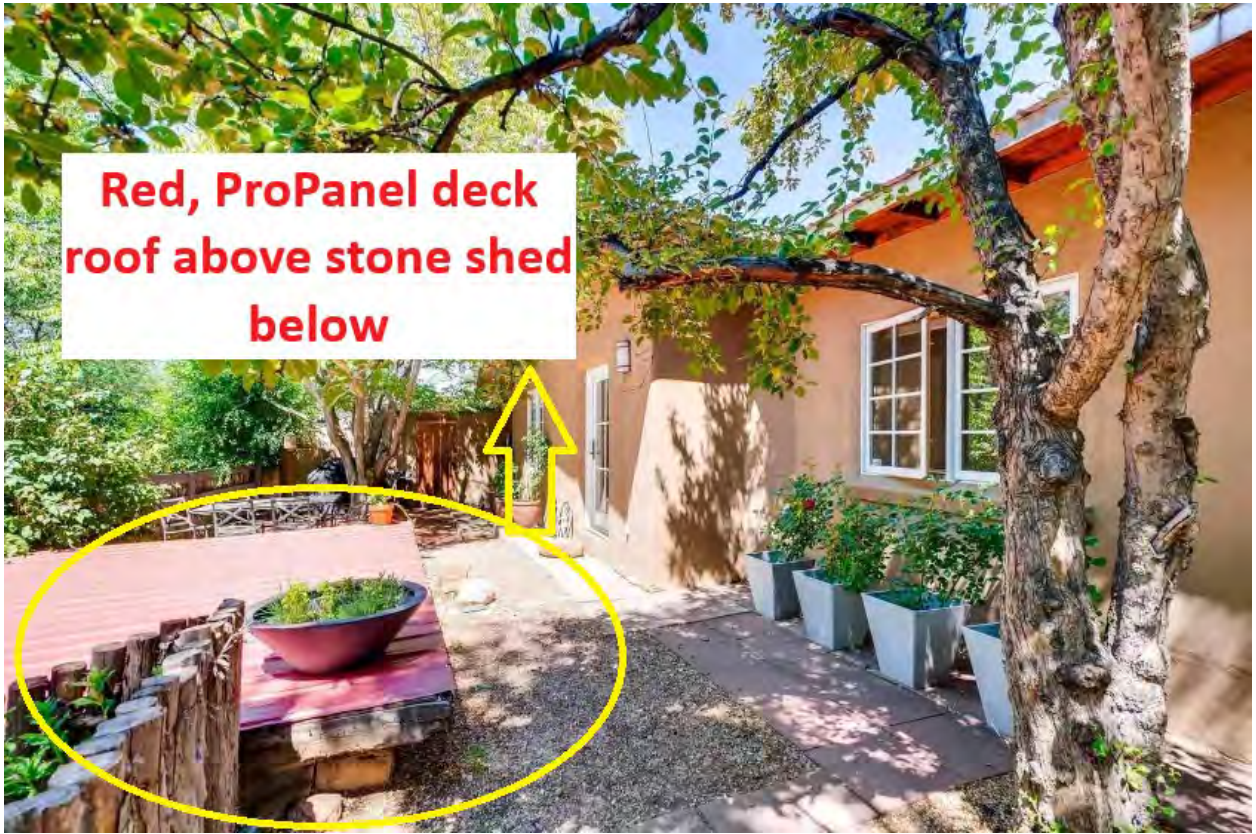
This is a picture of the south elevation from Zillow. This shows what the Backyard area looked like before Lisa Andree Falls took over ownership. The Red propanel material served as the stone shed's roof prior.
