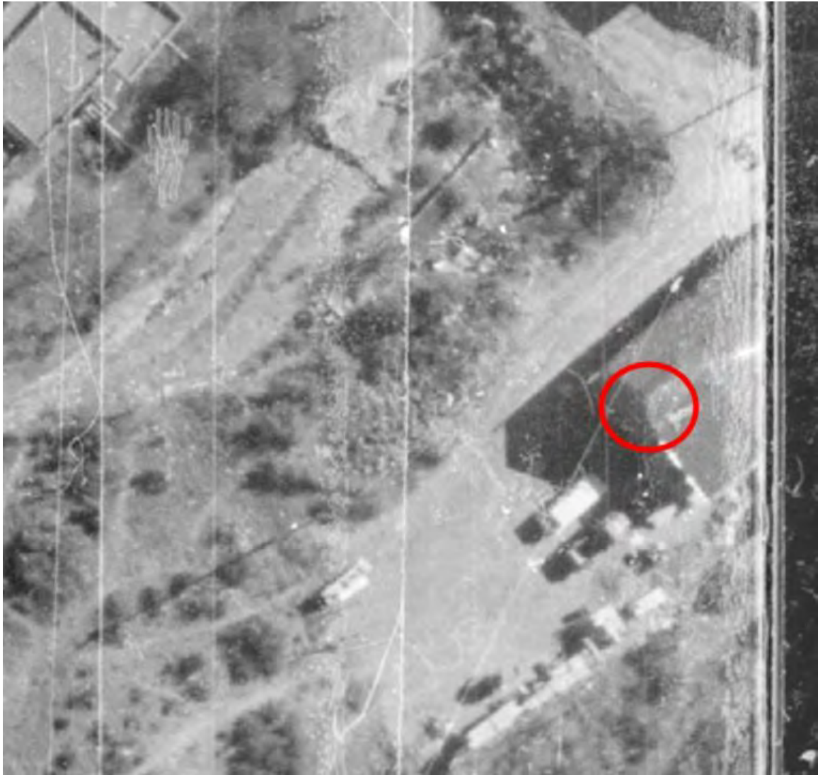
Figure 8: May 11, 1973, aerial photograph. Note the west connection has been simplified to a gable end (circle).
