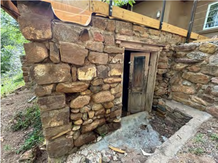
Figure 4: Exterior of the Shed
