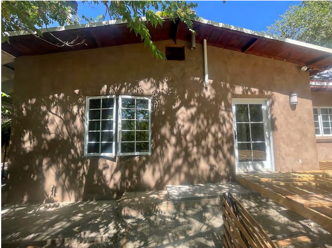
Photo 6: South elevation. Circa 1973-78 extension of west arm of historic C-shape plan. Camera facing north.
