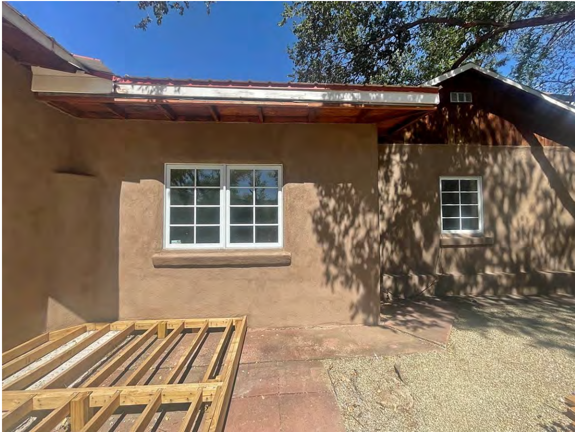
Photo 7: South elevation. Circa 1960-66 addition built across courtyard at center. Camera facing north.
