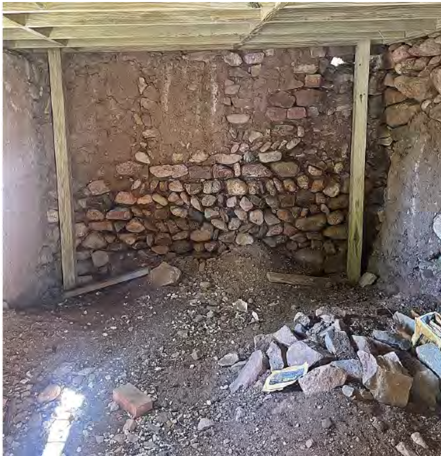
Figure 5: Stone shed structure interior
