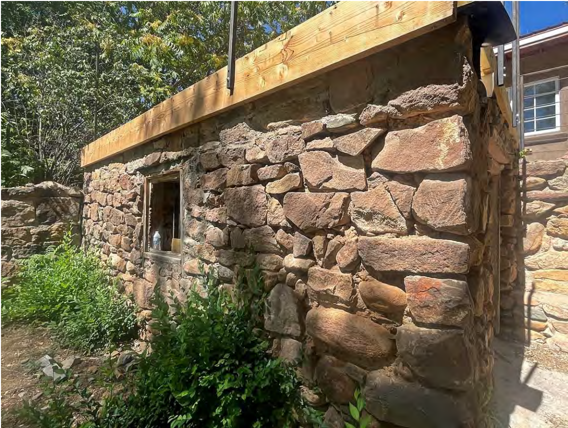
Photo 14: Stone structure. South elevation. Camera facing northwest.
