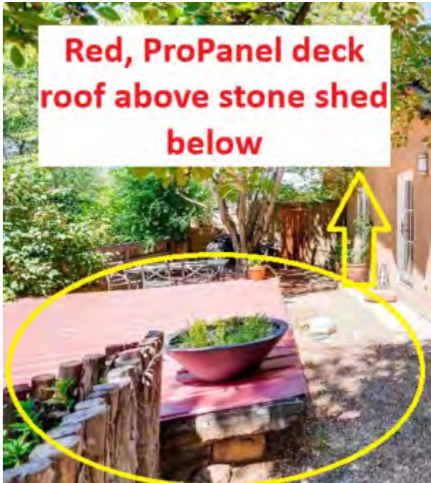
Figure 6: Previous red panel roof on the shed
