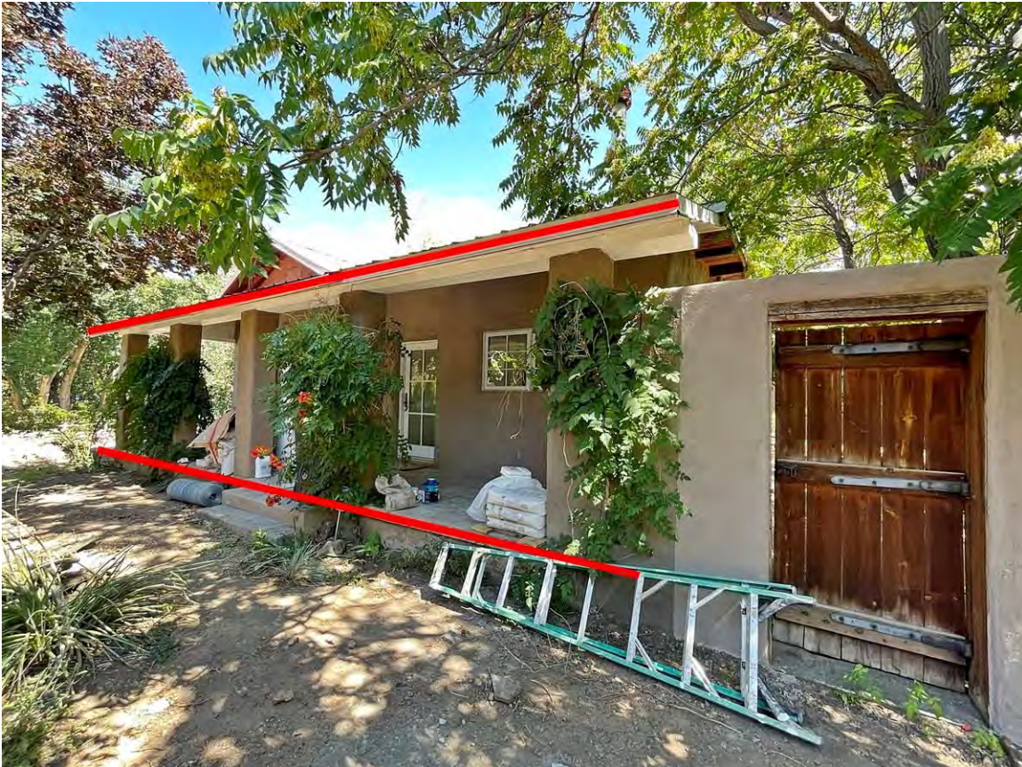
Photo 4: West elevation. Camera facing northeast. Craftsman-style porch (highlighted) postdates 1978.
