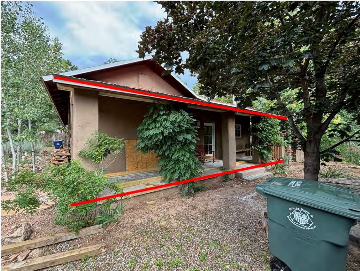
Photo 3: West elevation. Camera facing southeast. Craftsman-style porch (highlighted) postdates 1978. M. Kay, August 14, 2024.
