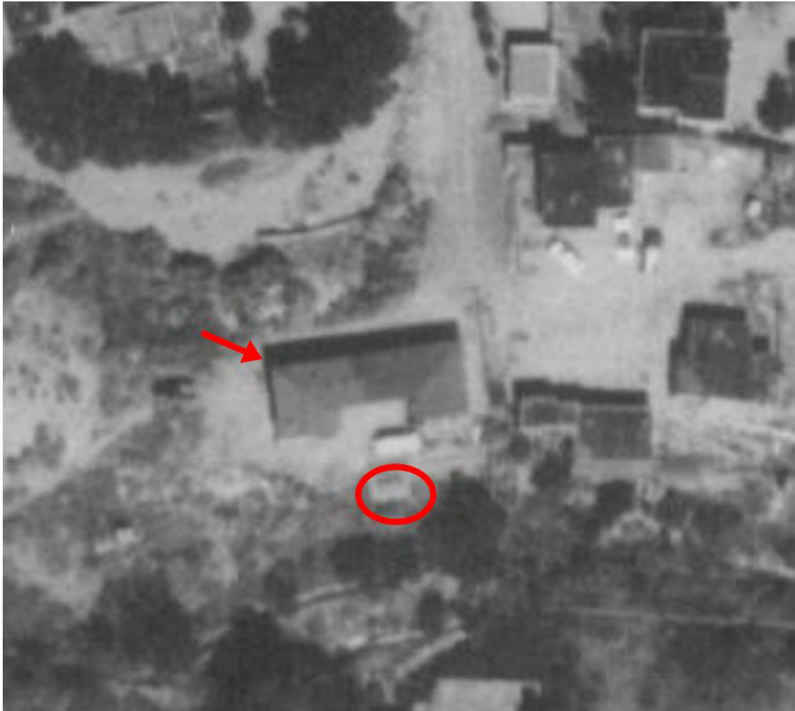
Figure 6: September 25, 1960, aerial photograph. Note hipped gable connection (arrow) and presence of a structure near the current day stone building (circle). Upper retaining wall and acequia are visible.
