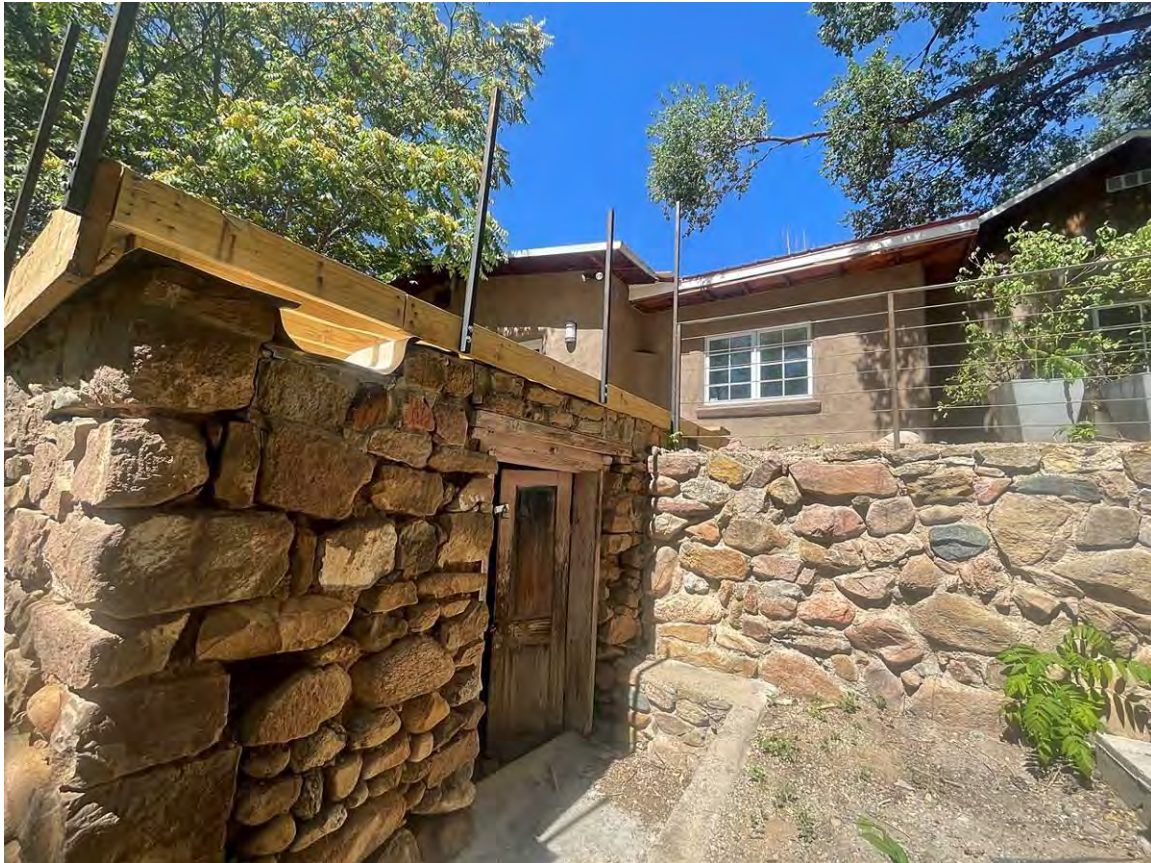
Photo 10: Stone structure (left) and upper retaining wall (right). Camera facing northwest.
