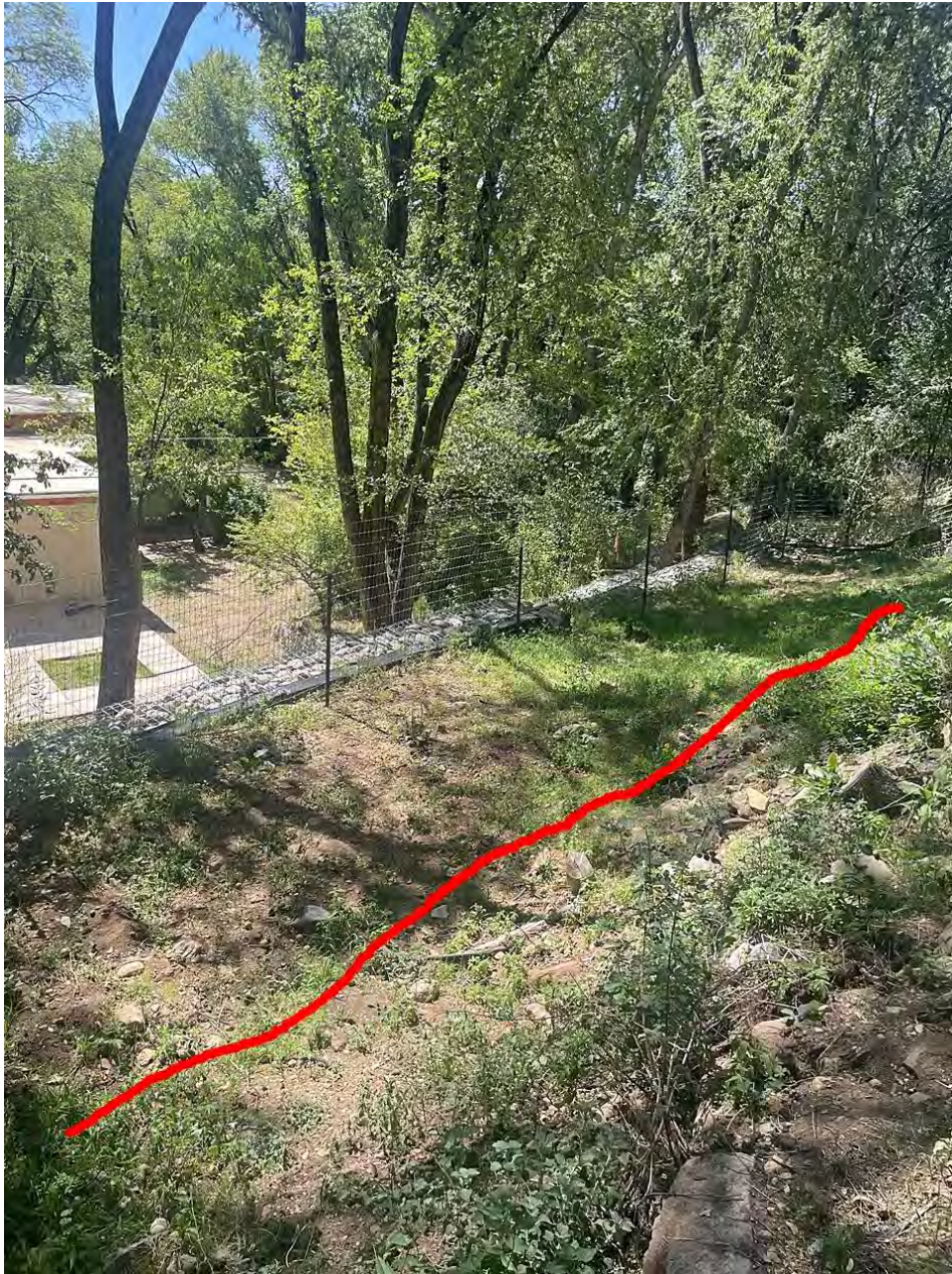
Photo 18: Remnant of Acequia de la Muralla or Ditch No 8. Camera facing southwest.
