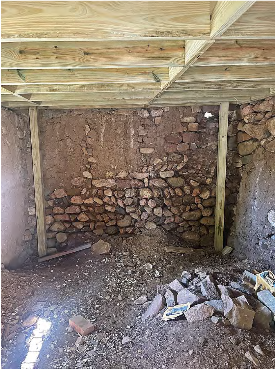
Photo 17: Stone structure. Interior. Camera facing west.
