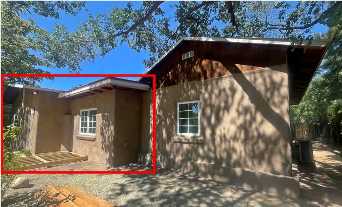
Photo 8: South elevation. The highlighted area represents 1960s and '70s additions filling in the historic patio area. Camera facing northwest.
