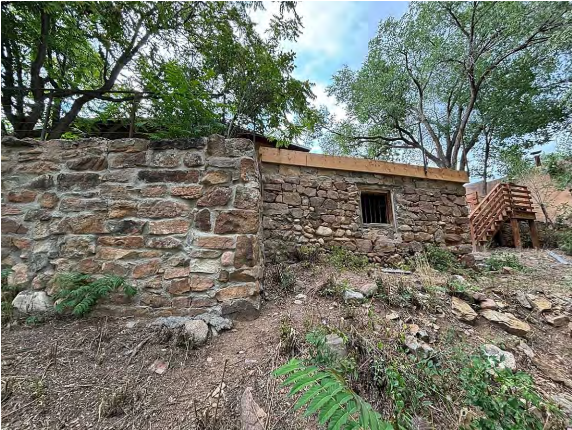
Photo 11: Upper retaining wall (left) and stone structure (right). Camera facing northeast. M. Kay, August 14, 2024.
