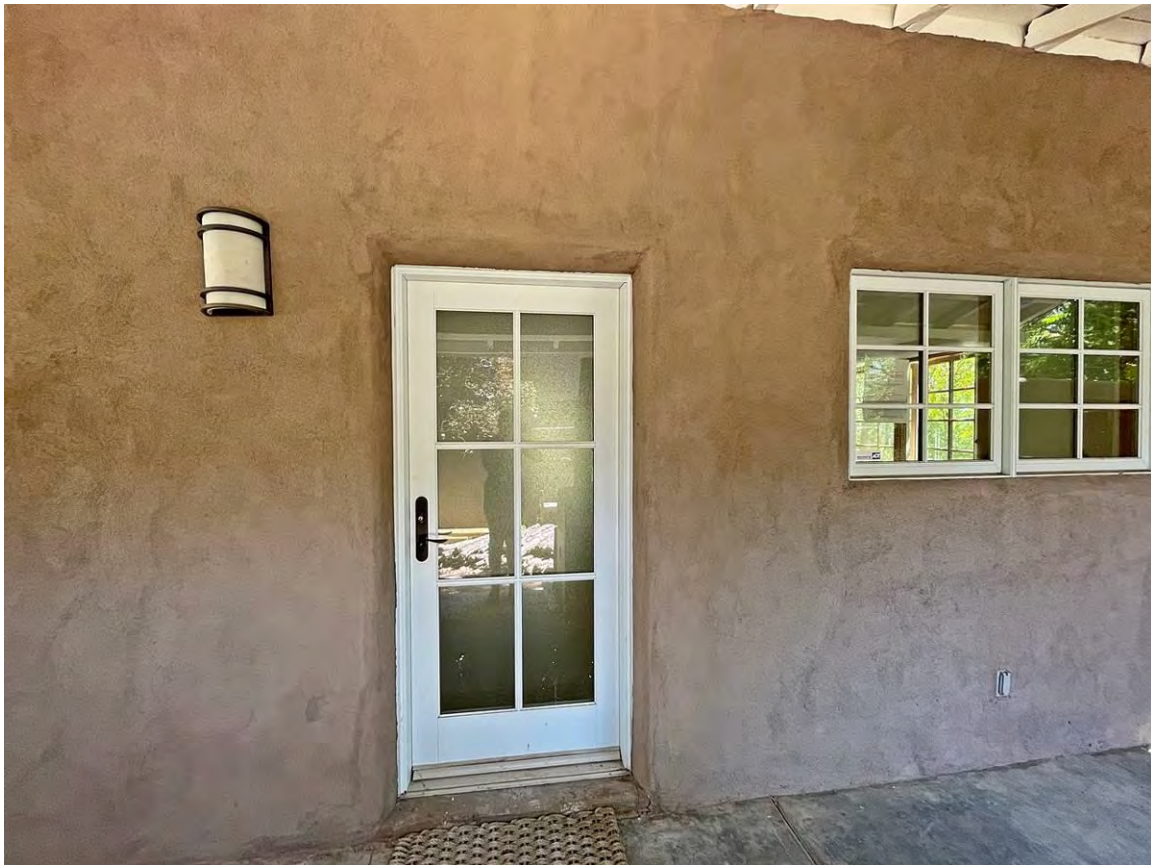
Photo 5: West elevation. Entry and fenestration. Camera facing southeast.
