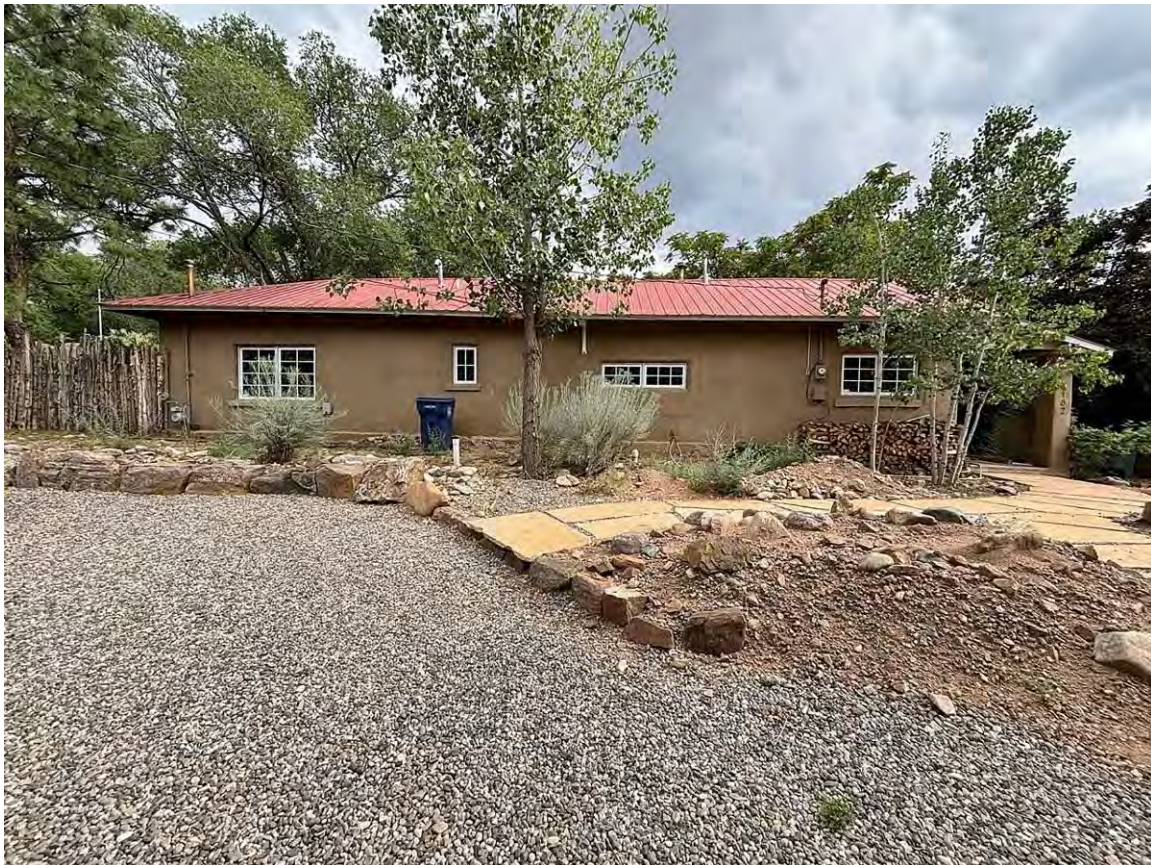
Photo 2: North elevation. Camera facing south. M. Kay, August 14, 2024.
