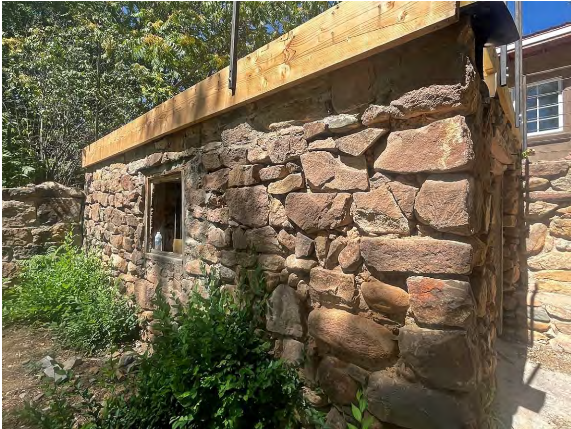
Photo 14: Stone structure. South elevation. Camera facing northwest.
