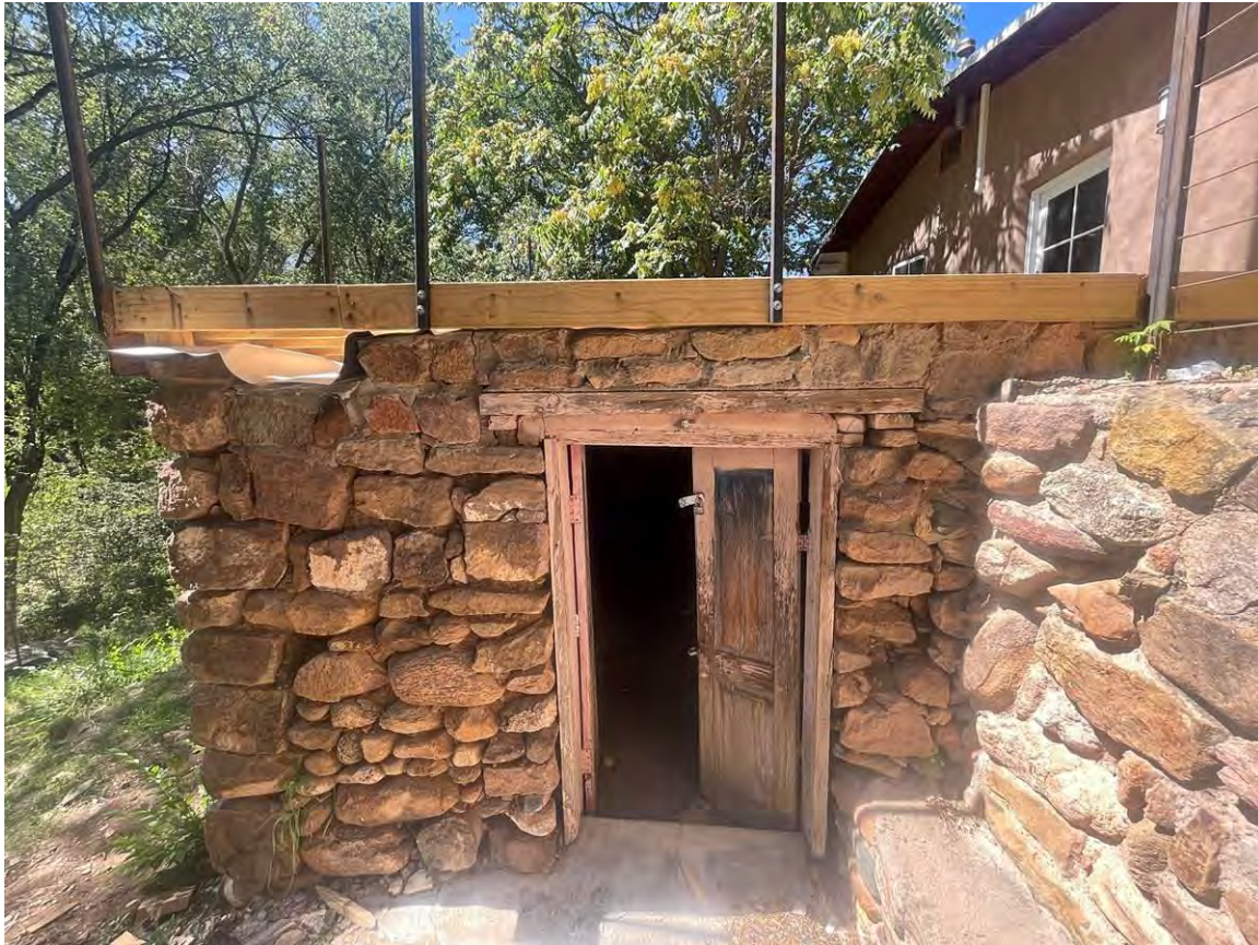
Photo 13: Stone structure. East elevation. Camera facing west.
