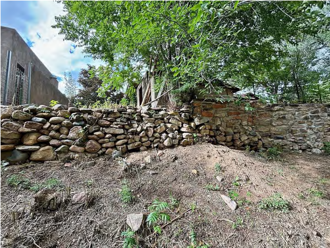
Photo 12: Upper retaining wall at west end. Camera facing north. M. Kay, August 14, 2024.
