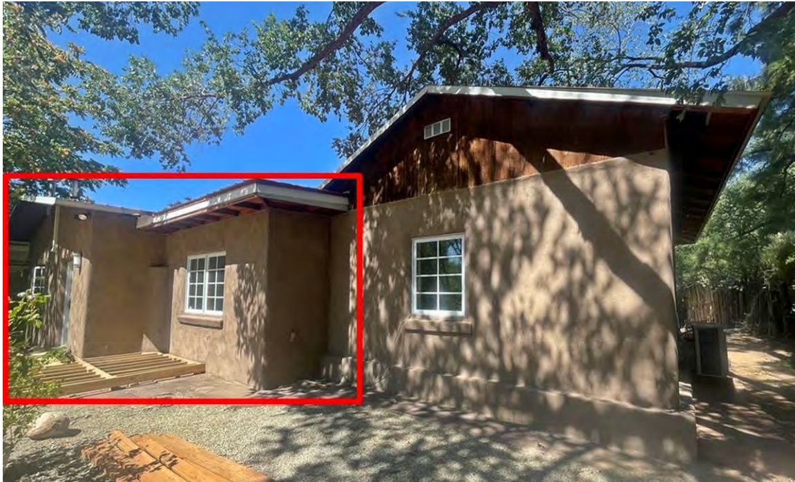
Photo 8: South elevation. The highlighted area represents 1960s and '70s additions filling in the historic patio area. Camera facing northwest.
