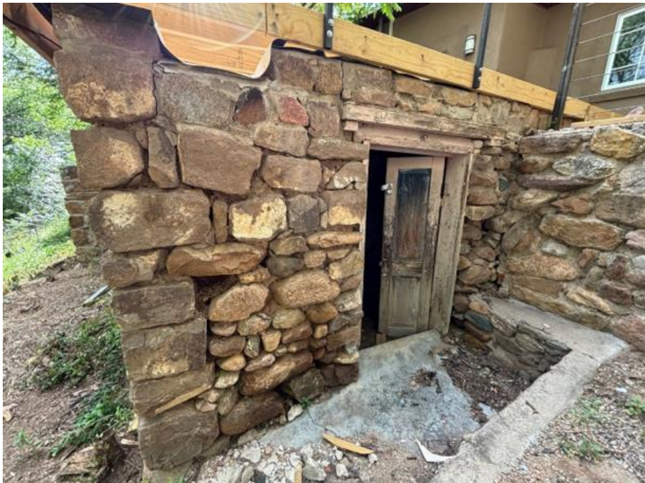
Figure 2: Exterior of the Shed
