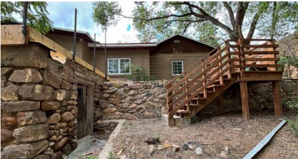
Figure 3: Stairs constructed on yardwall and deck as roof on stone structure.
