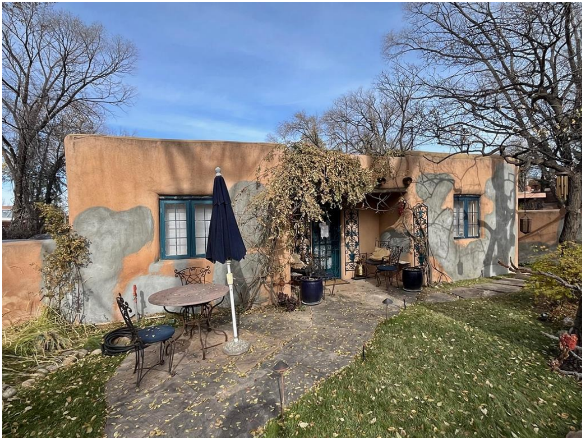
Photo 2: South (front) elevation. Camera facing northeast.
