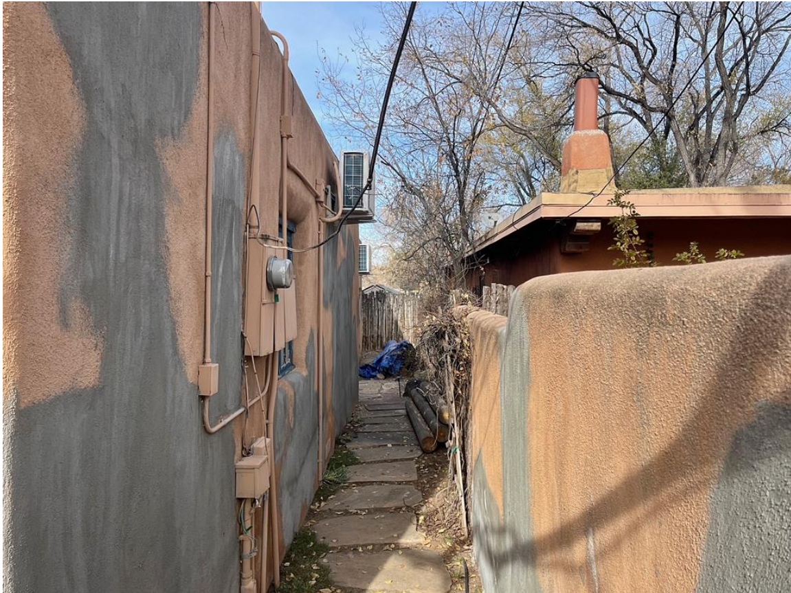
Photo 6: East elevation oblique. Camera facing north.
