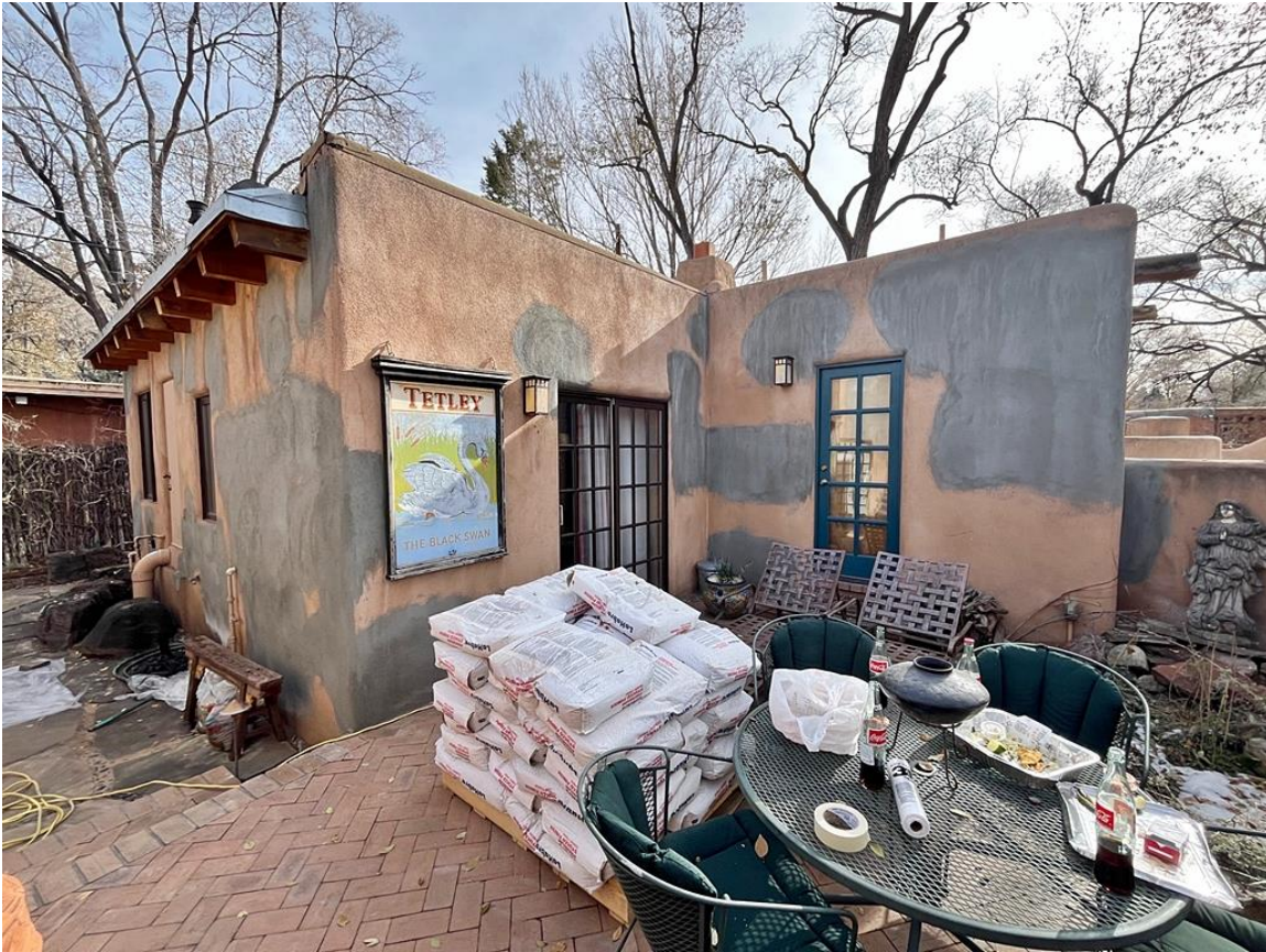
Photo 11: Northwest (patio) elevation. Camera facing southeast.
