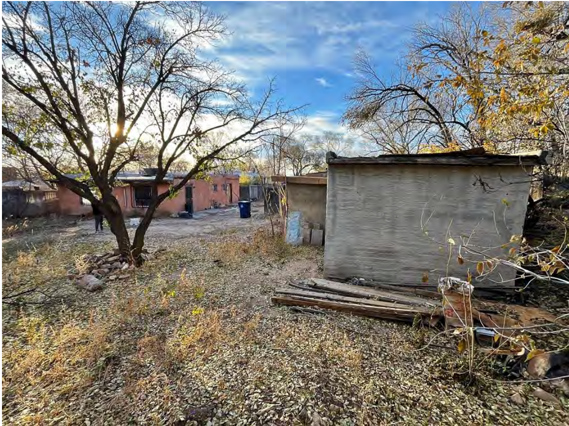
Photo 3: View of property facing southwest. Non-historic shop at foreground right.
