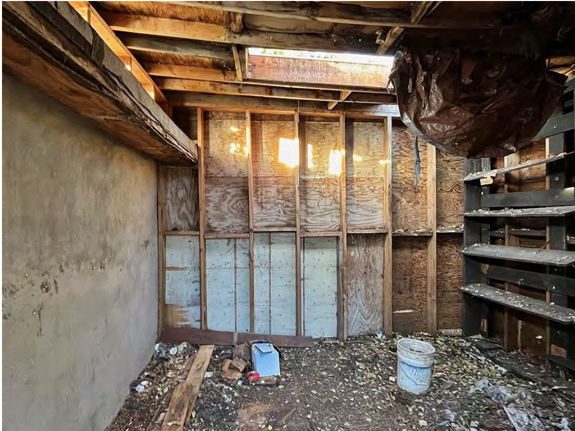
Photo 26: Photo 25: Shop. Addition, interior. Camera facing north.
