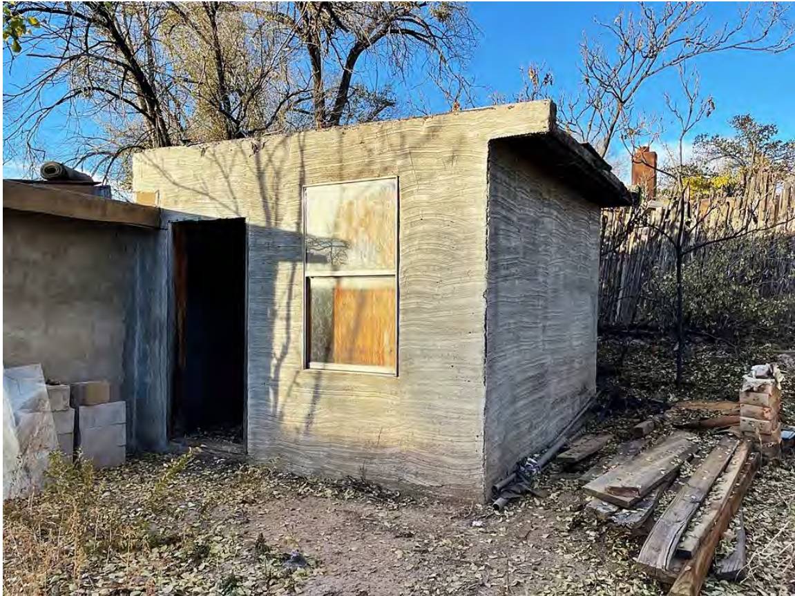
Photo 25: Shop. Addition. Camera facing northwest.
