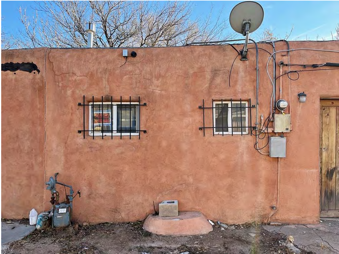
Photo 7: North elevation fenestration representing the kitchen (left) and bathroom (right) of the northeast room of the original core. Camera facing south.
