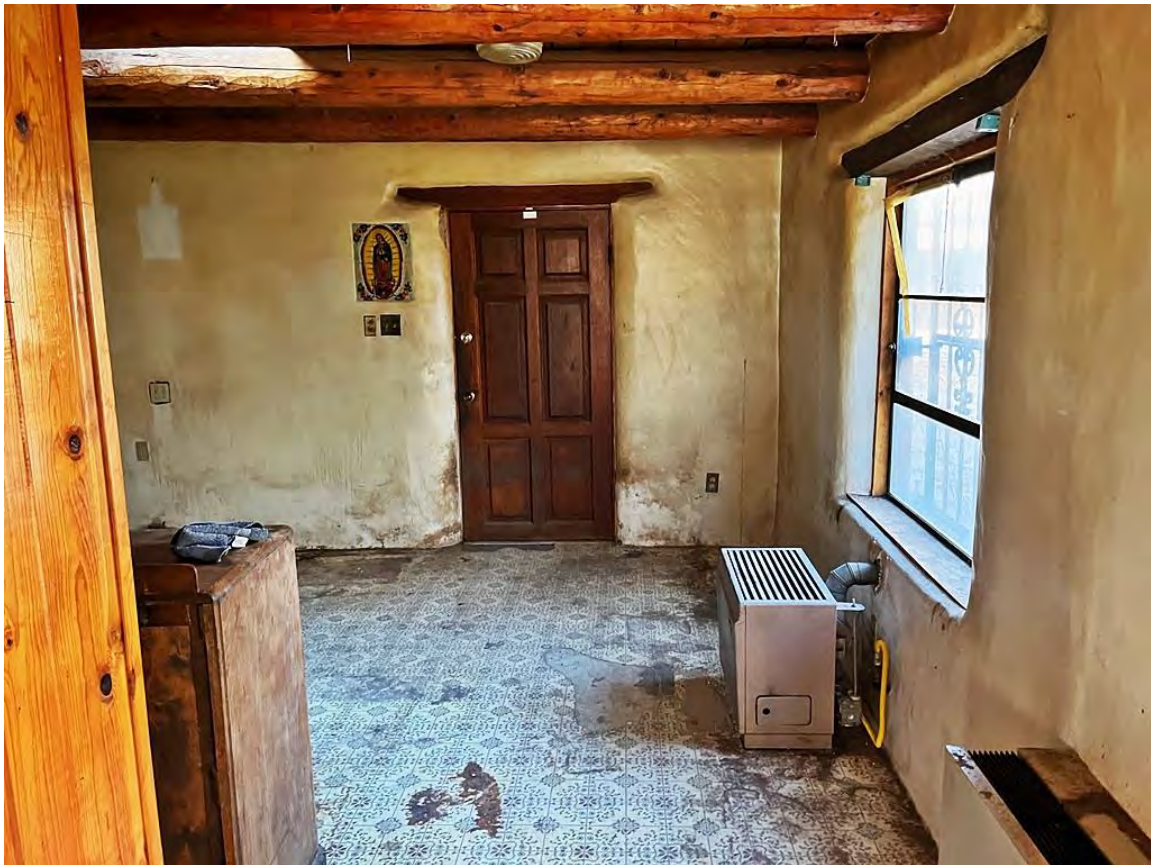
Photo 22: 1980s addition. Camera facing north.
