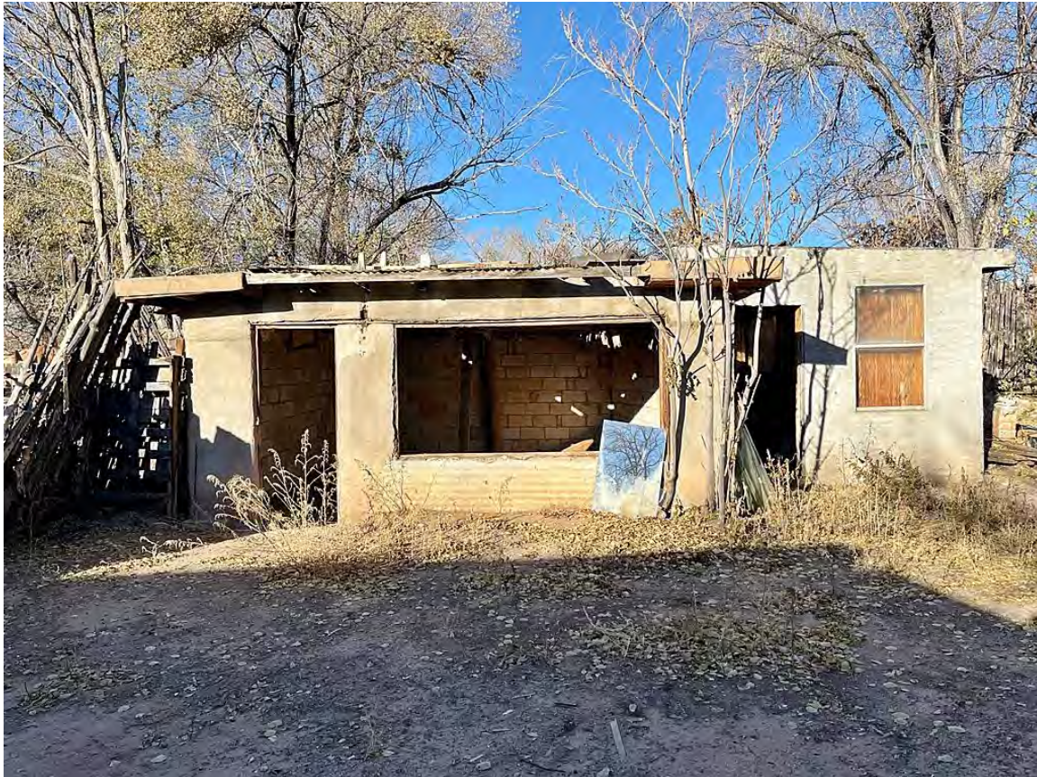
Photo 23: Shop. South elevation. Camera facing north.
