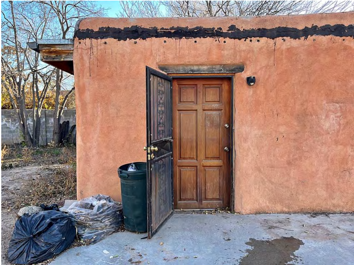
Photo 8: North elevation at east end addition. Camera facing south.
