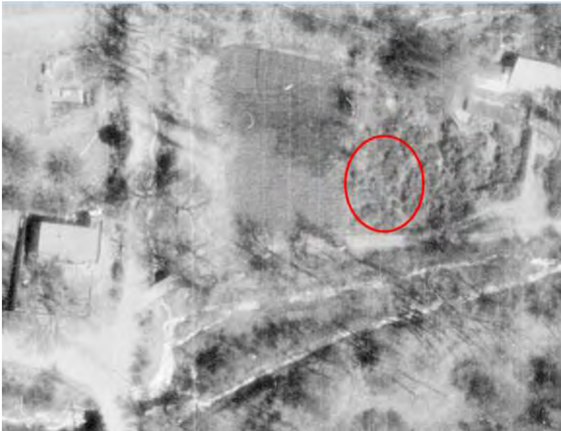
Figure 9: May 5, 1966, aerial photograph. Approximate location of future house circled.
