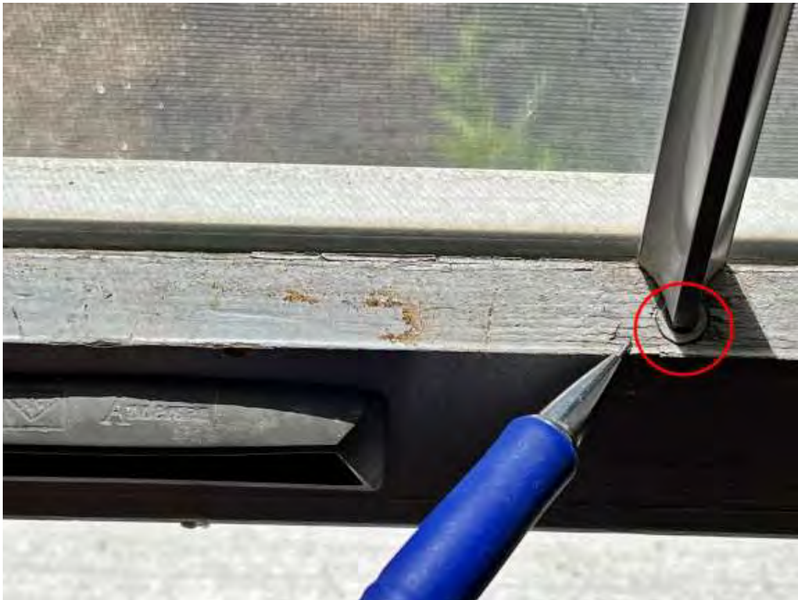
Photo 5: Andersen Narroline windows showing snap-in socket. Camera facing down. August 3, 2023.
