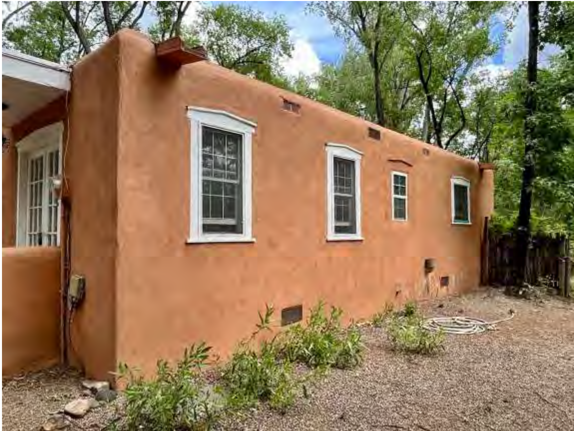
Photo 10: West elevation. Camera facing southeast.
