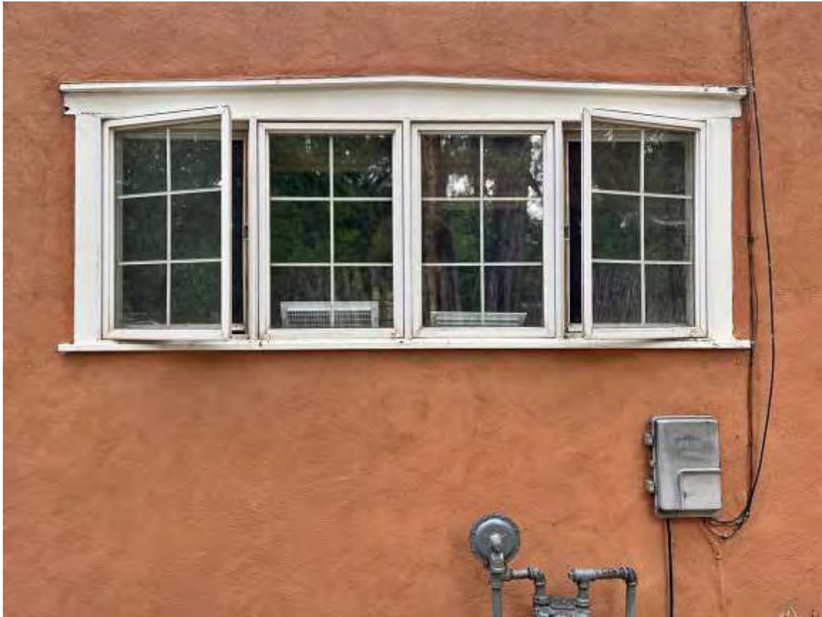
Photo 8: East elevation, casement windows. Camera facing west.
