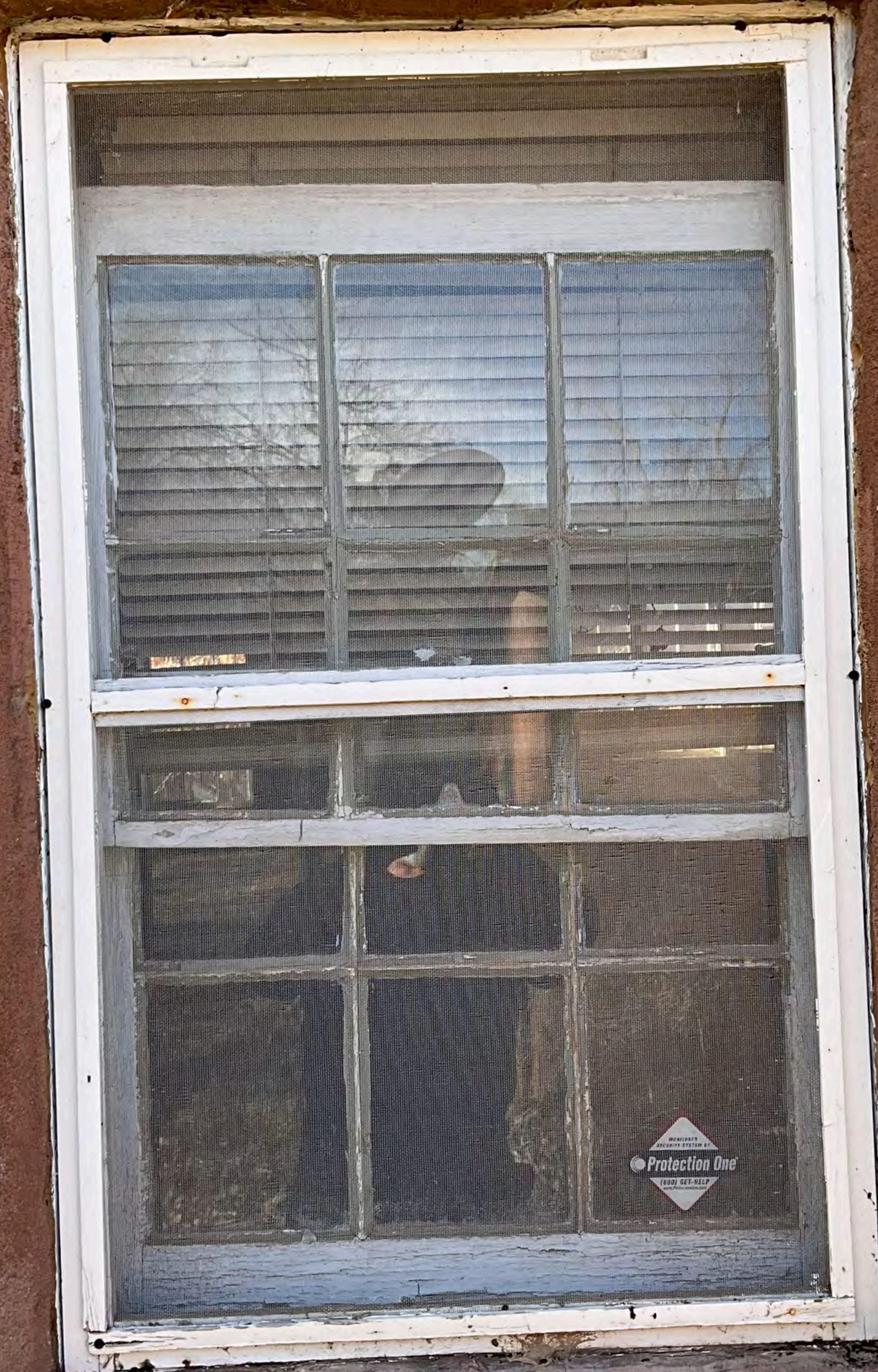
East Elevation Window D
