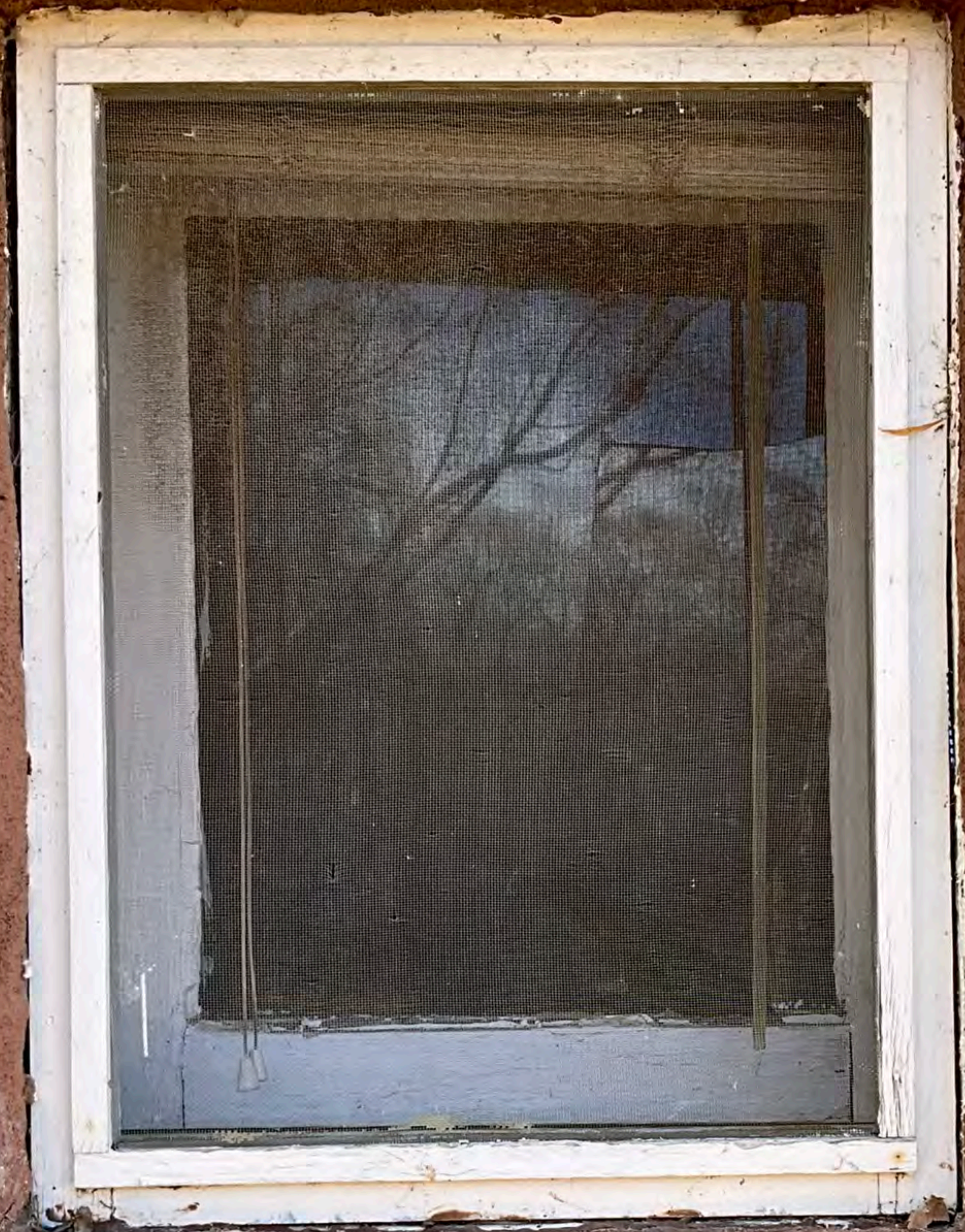
East Elevation Window C
