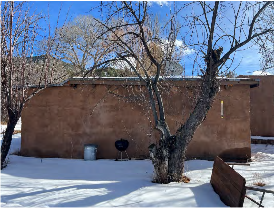
North Side – Shed / Garage Rear Elevation
