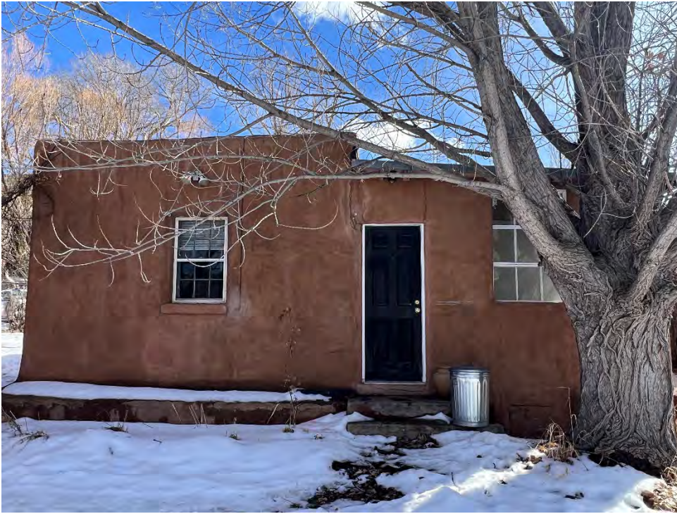
North Side – Residence Rear Elevation
