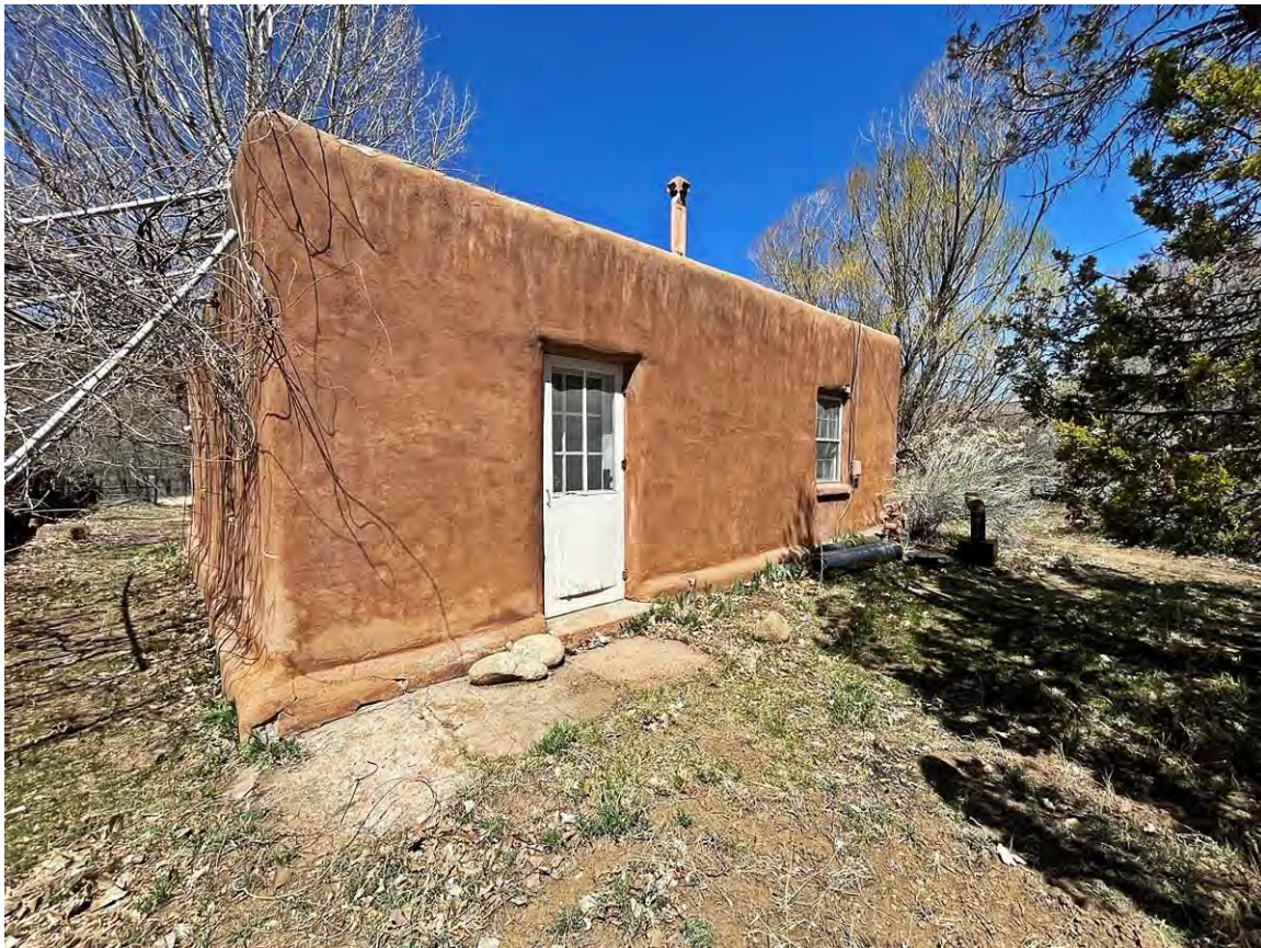
Photo 2: South elevation. Camera facing northeast.
