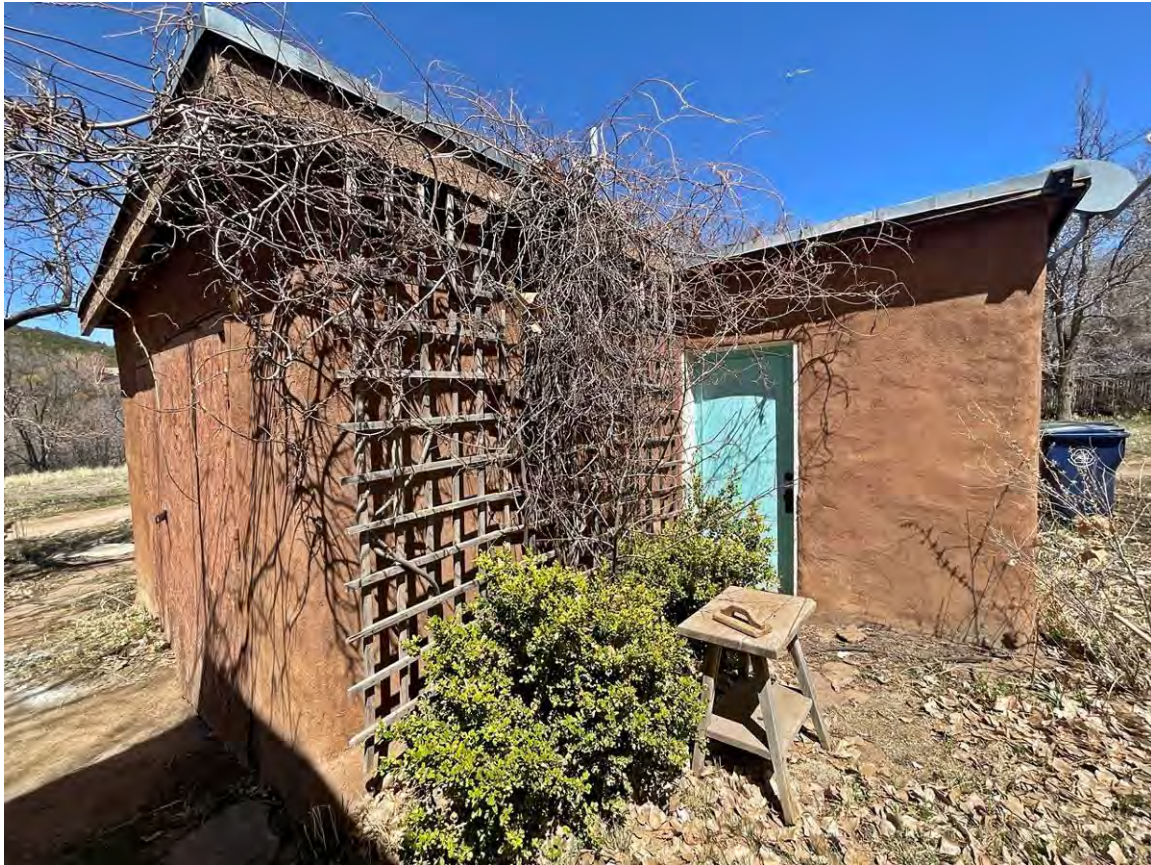
Photo 9: West elevation. Camera facing northeast.
