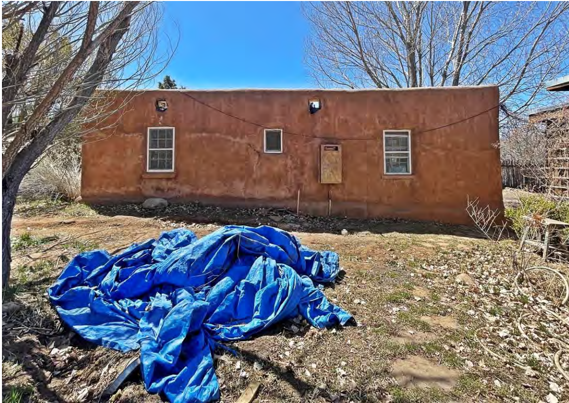
Photo 4: East elevation. Camera facing west.
