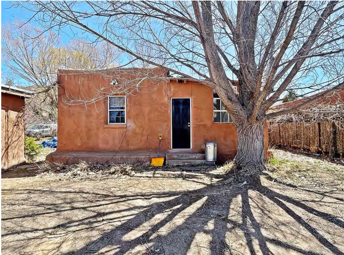
Photo 5: North elevation. Camera facing south.
