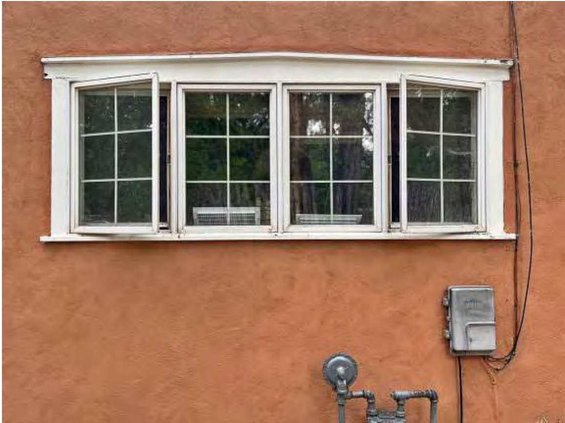
Photo 8: East elevation, casement windows. Camera facing west.
