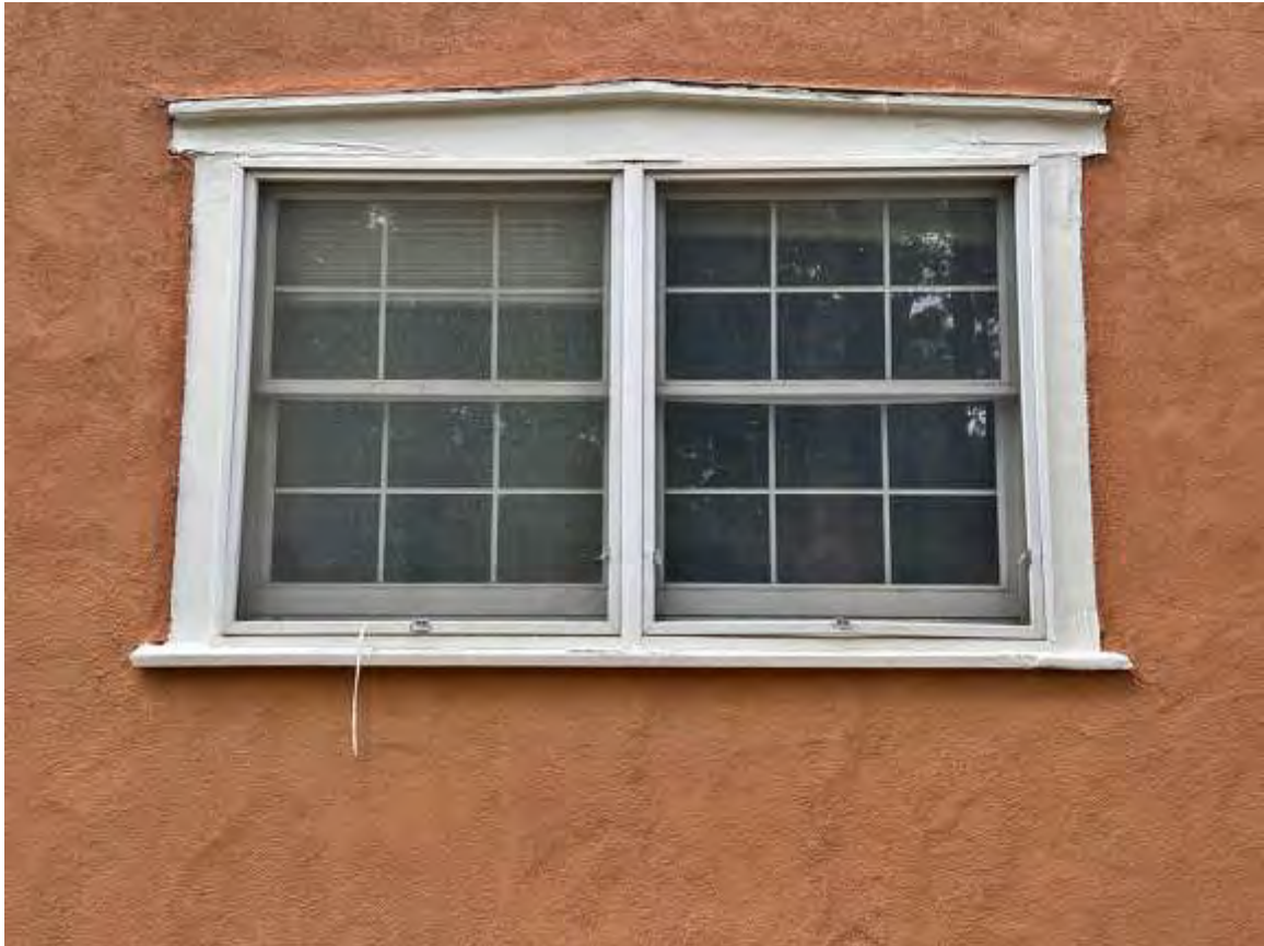
Photo 4: Andersen Narroline windows. Front façade. Camera facing north.
