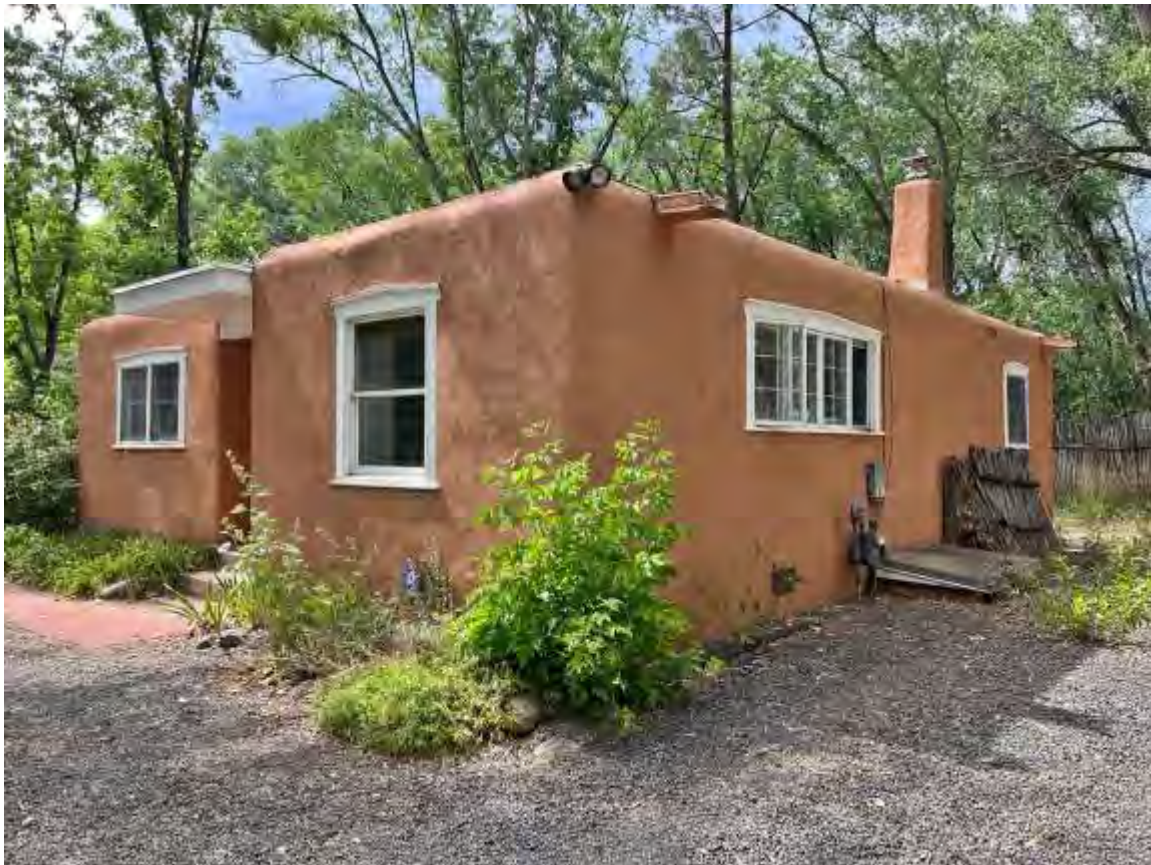
Photo 7: South and east elevations. Camera facing northwest.
