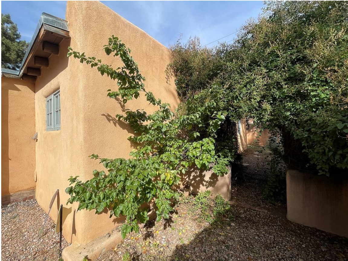
Photo 7: South elevation, at southwest corner. Enclosed porch at left. Camera facing northeast.
