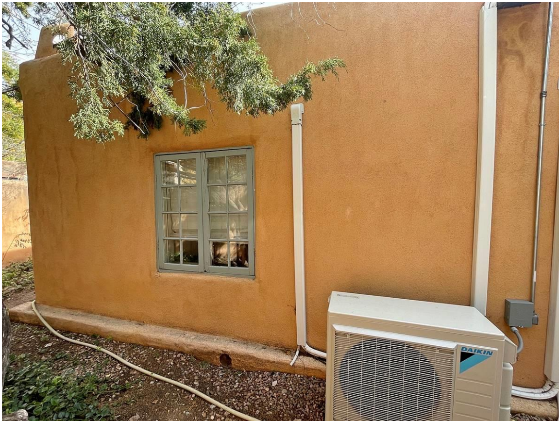
Photo 11: North elevation, northeast corner. Camera facing southeast.
