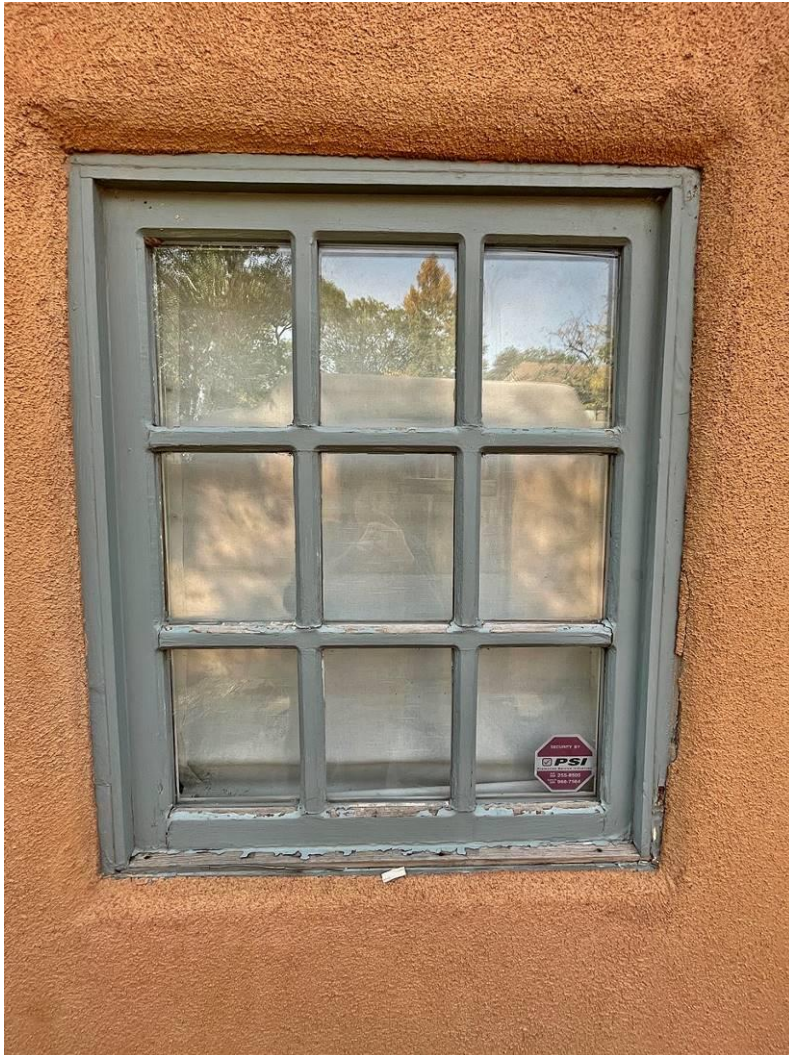
Photo 4: East elevation, portal enclosure. Non-historic window. Camera facing southeast.
