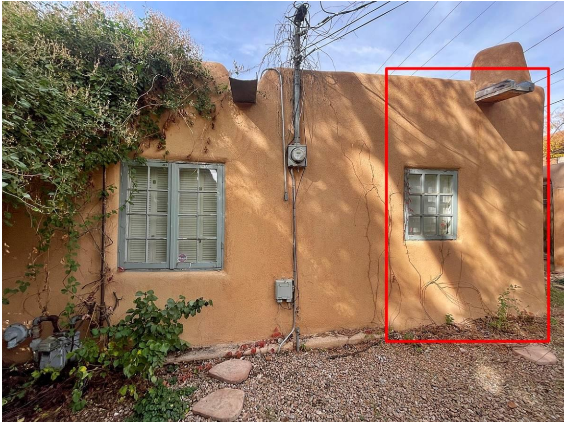
Photo 5: South elevation, east end. 1970s portal enclosure highlighted. Camera facing northeast.
