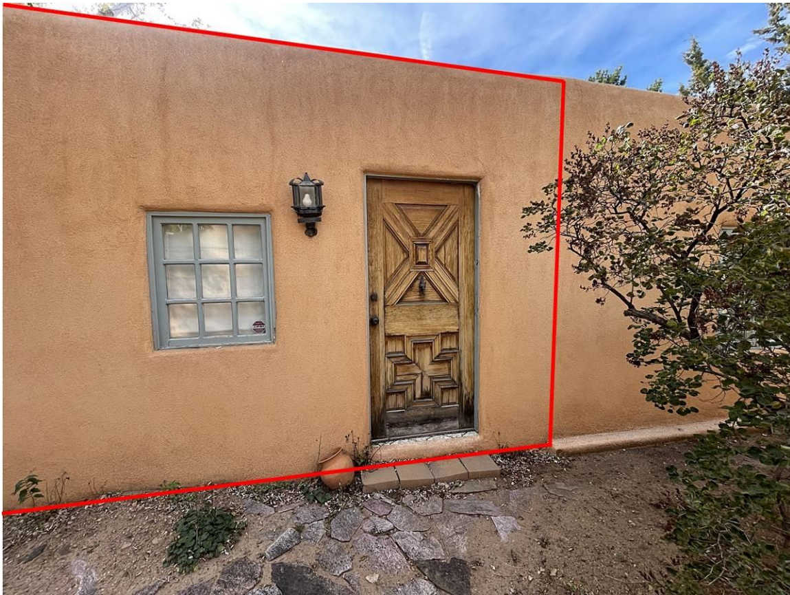
Photo 3: East elevation, south end. 1970s portal enclosure highlighted. Camera facing northwest.
