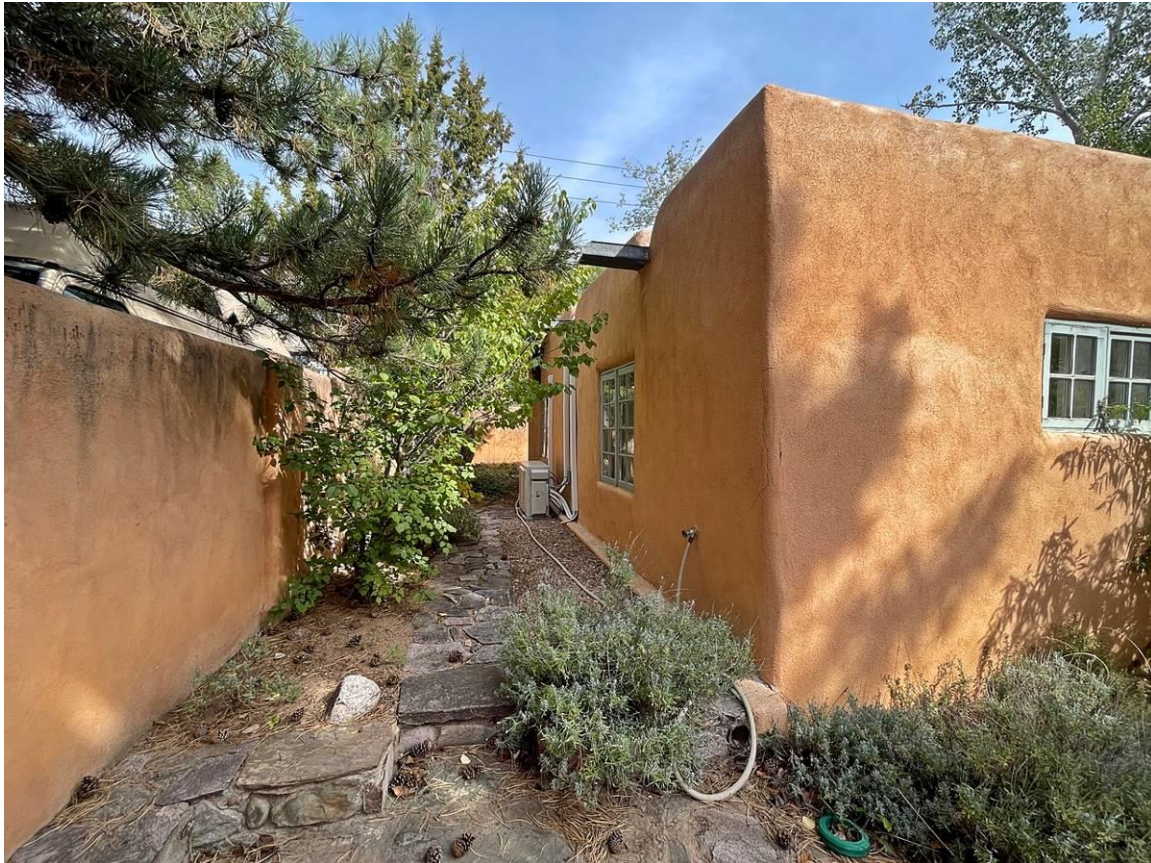
Photo 9: North elevation. Camera facing east.
