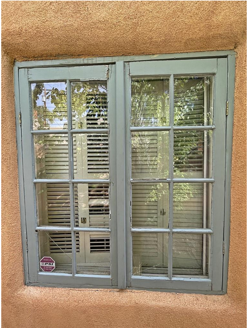
Photo 10: North elevation. Older casement windows.
