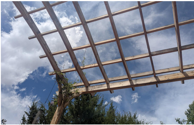
EXISTING WOODEN PERGOLA VIEW 1
