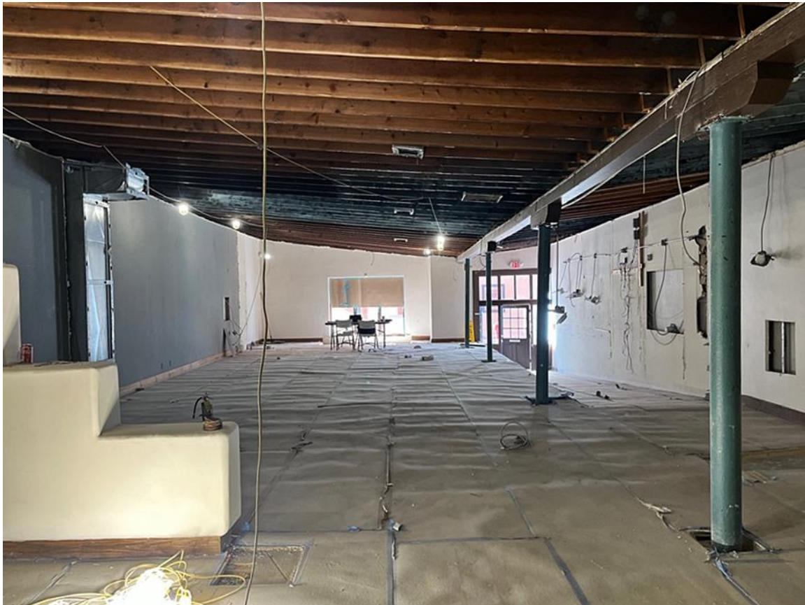
Photo 11: Interior. Camera facing south. December 2, 2025.
