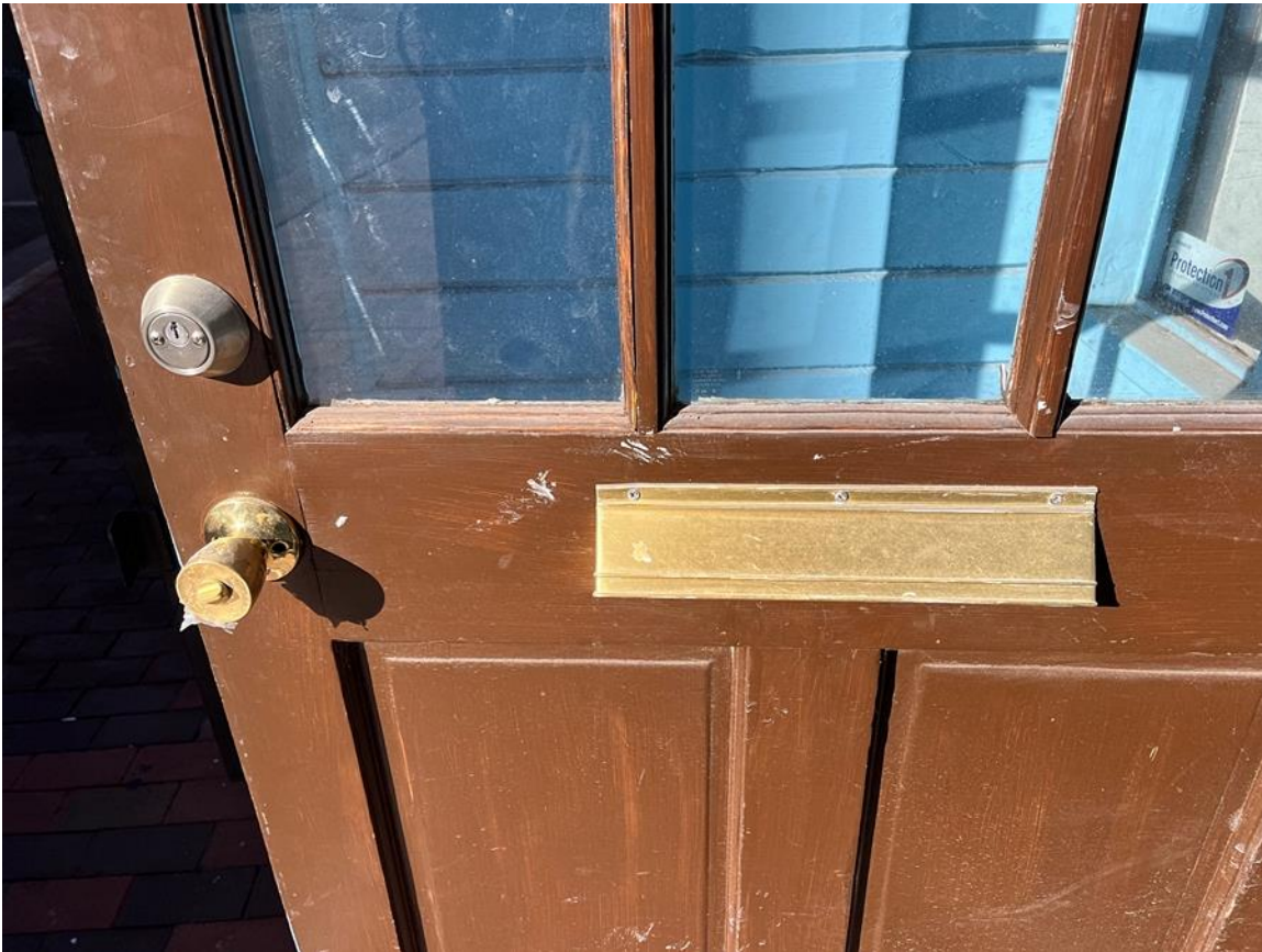
Photo 4: Entry door. Camera facing down and west. December 2, 2025.
