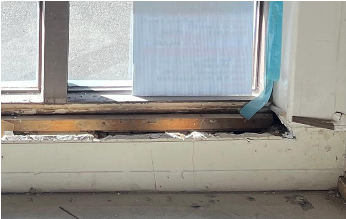
Photo 9: Display window from interior. Camera facing south. December 2, 2025.
