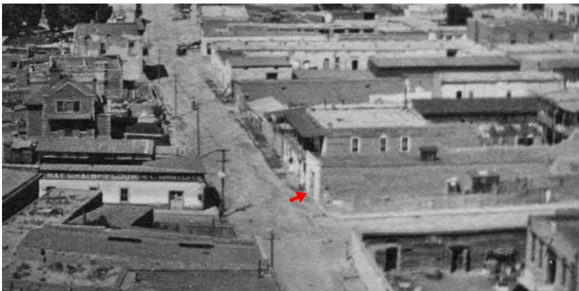
Figure 4: Portion of c.1909 – 1910 view of Water Street, taken from power plant smokestack. Large wood entry to building indicated by arrow.
