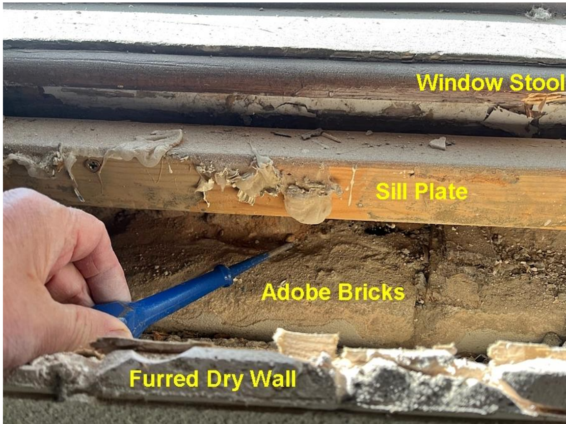
Photo 10: Detail of display window construction from interior. Camera facing down. December 2, 2025.
