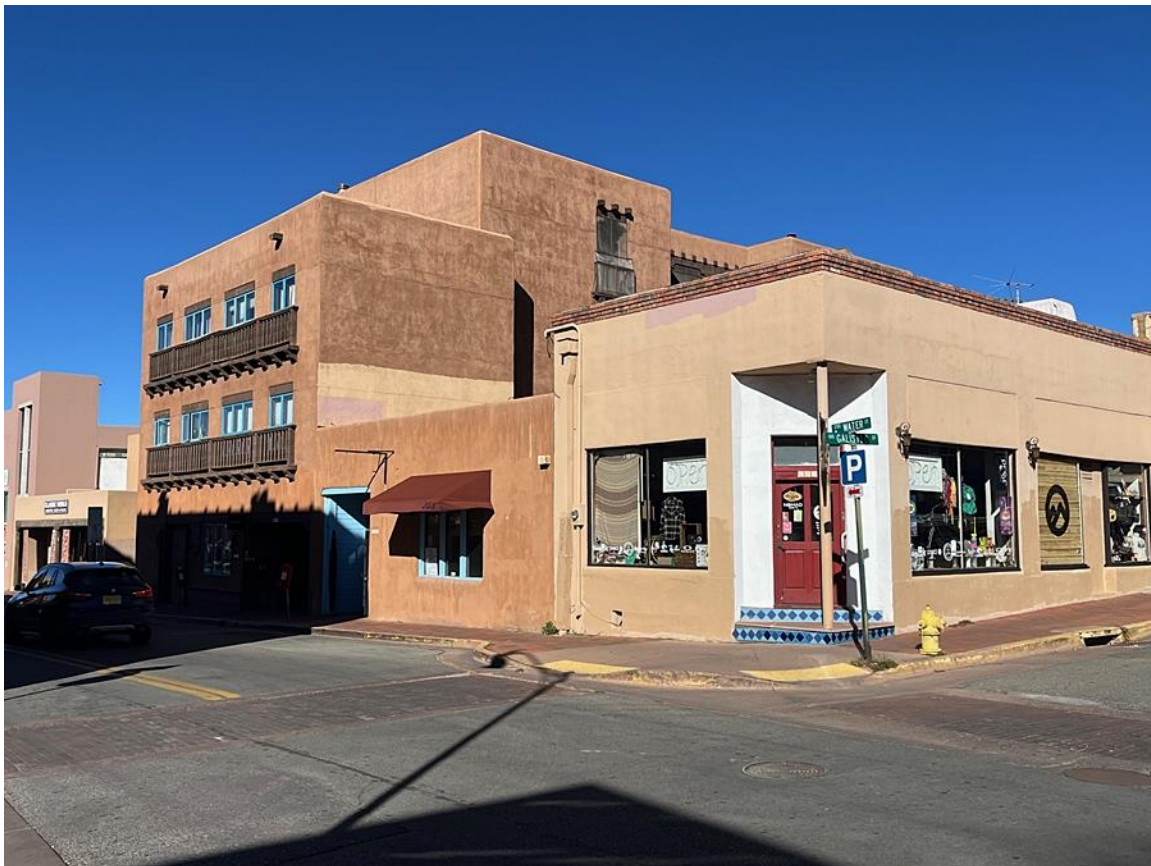
Photo 2: Setting. Camera facing northwest. December 2, 2025.
