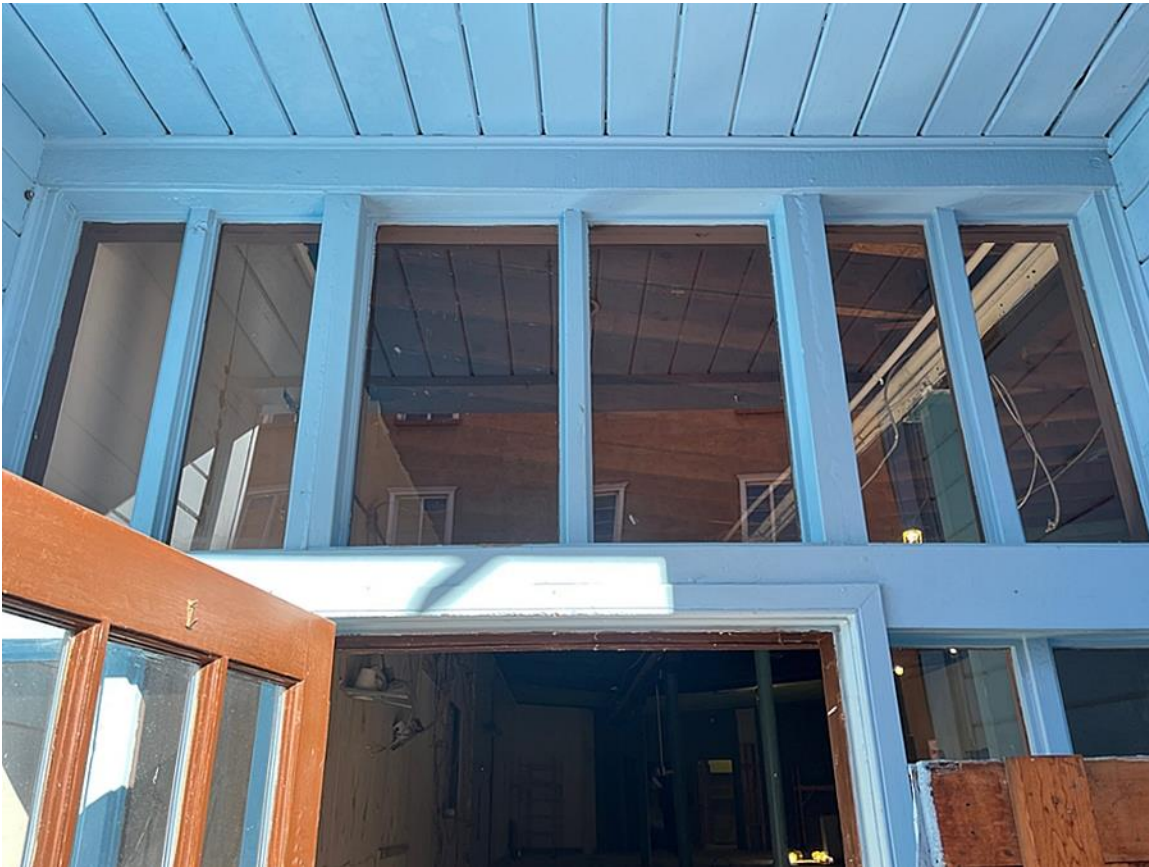
Photo 6: Transom. Camera facing up. December 2, 2025.
