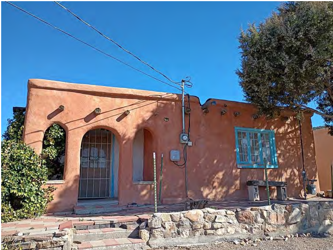
Photo 3: South (front) façade. Camera facing north.
