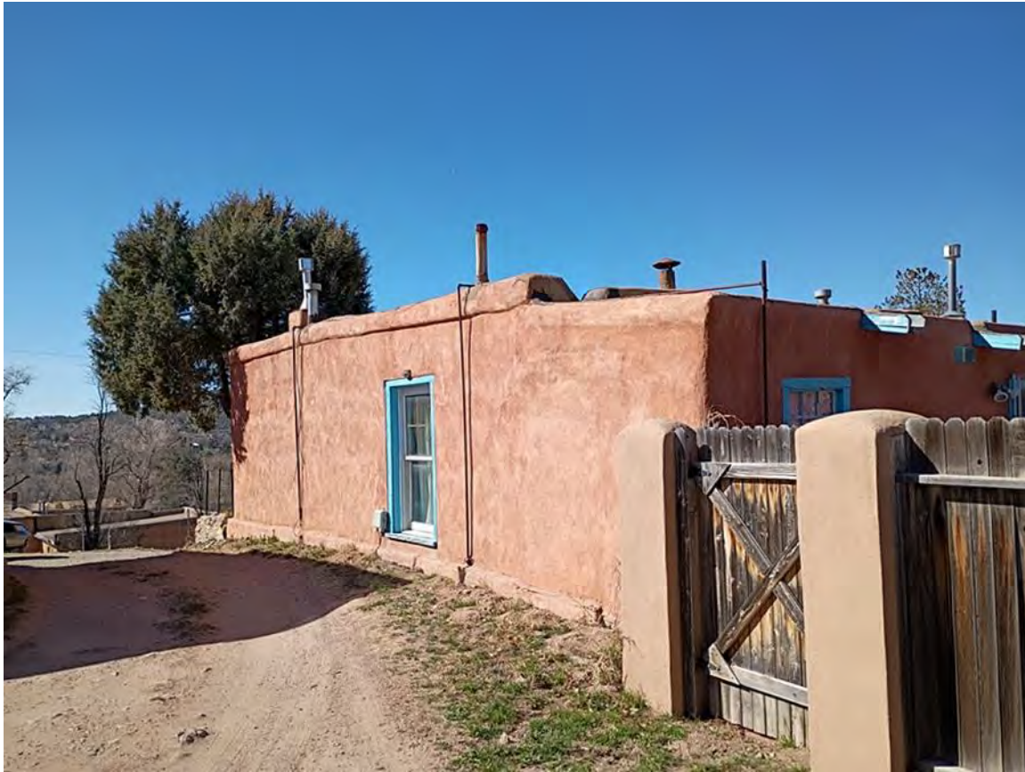
Photo 7: East elevation. Camera facing northwest.
