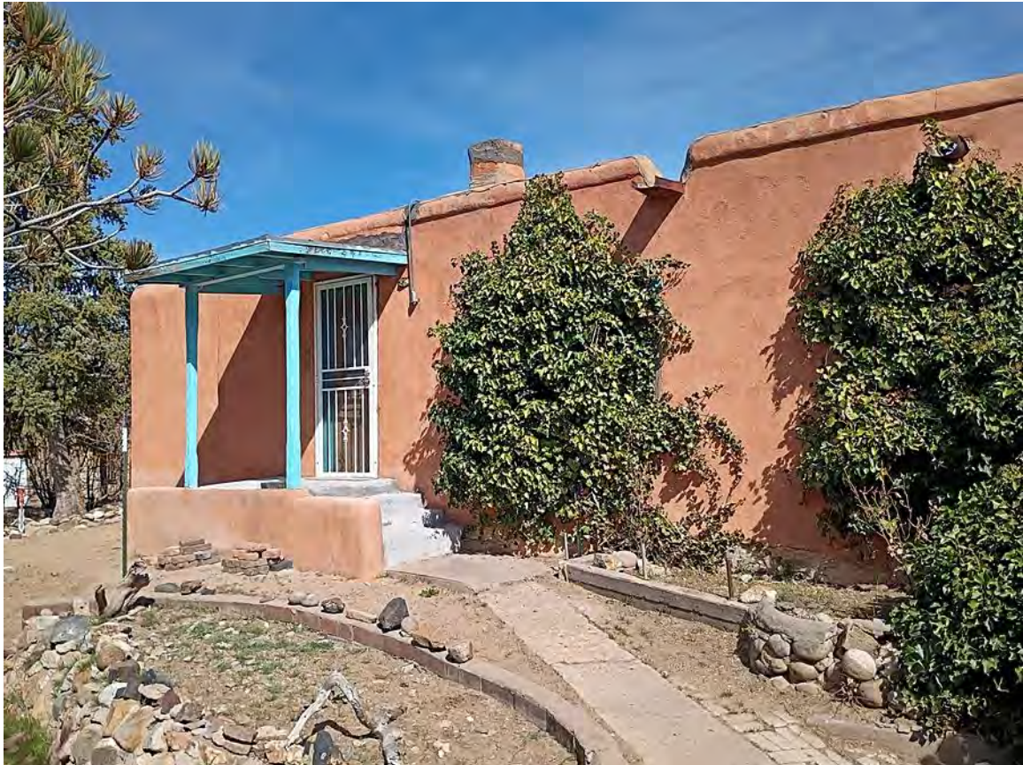
Photo 5: West elevation. Camera facing northeast.
