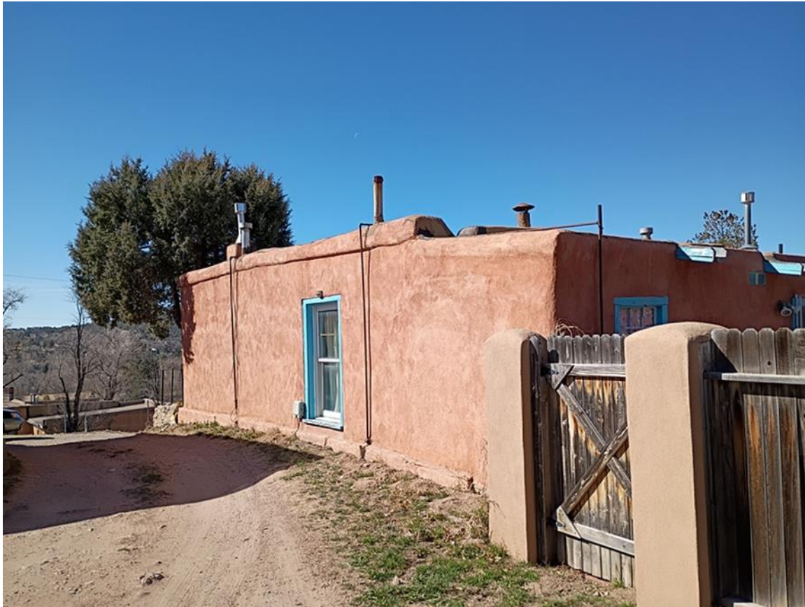
Photo 7: East elevation. Camera facing northwest.
