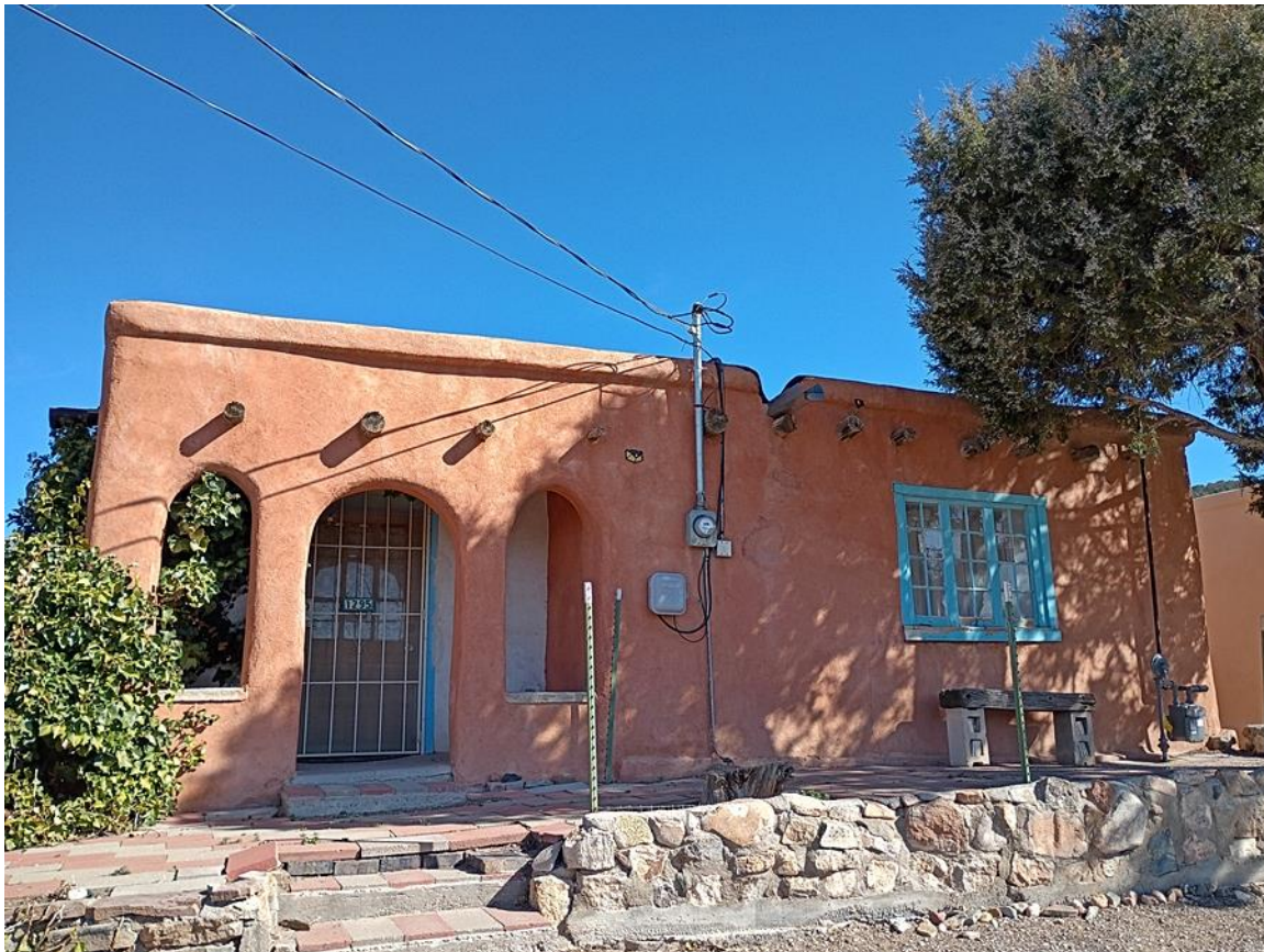
Photo 3: South (front) façade. Camera facing north.
