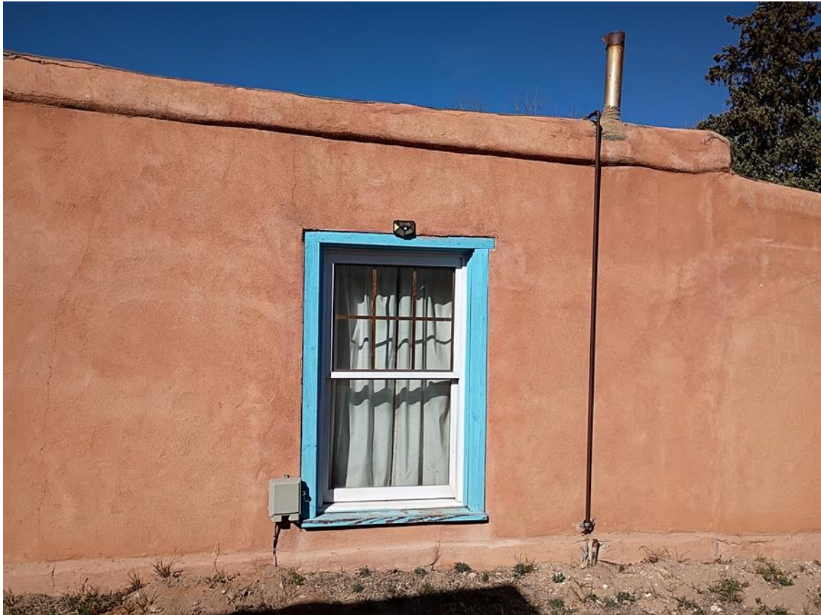
Photo 8: East elevation. Window detail. Camera facing west.
