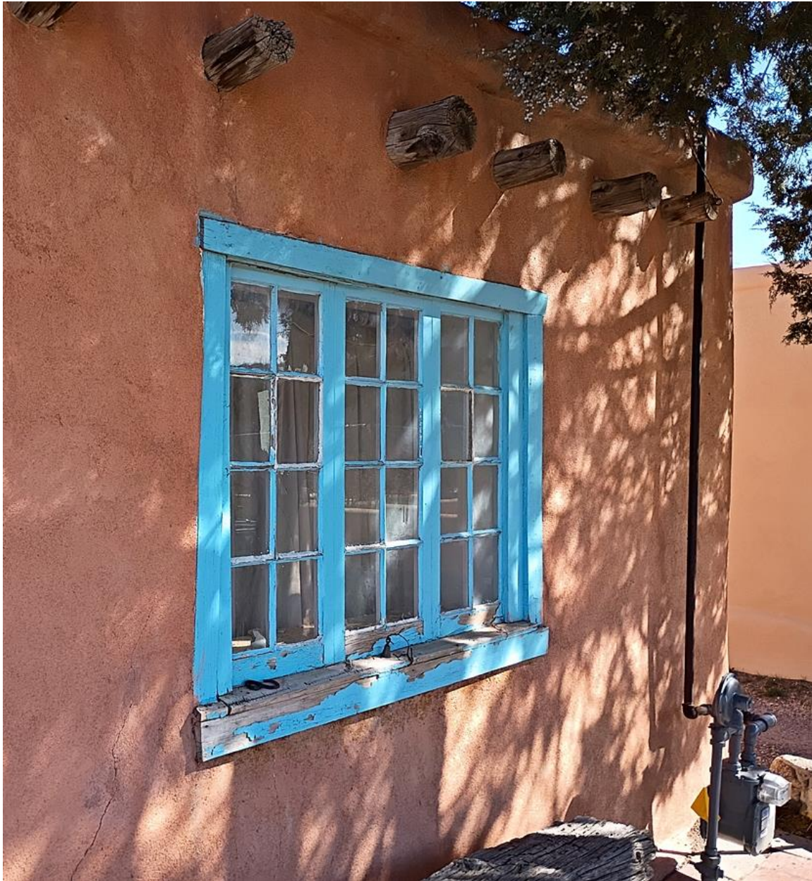
Photo 4: South (front) façade. Window detail. Camera facing northeast.
