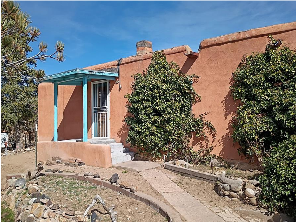
Photo 5: West elevation. Camera facing northeast.
