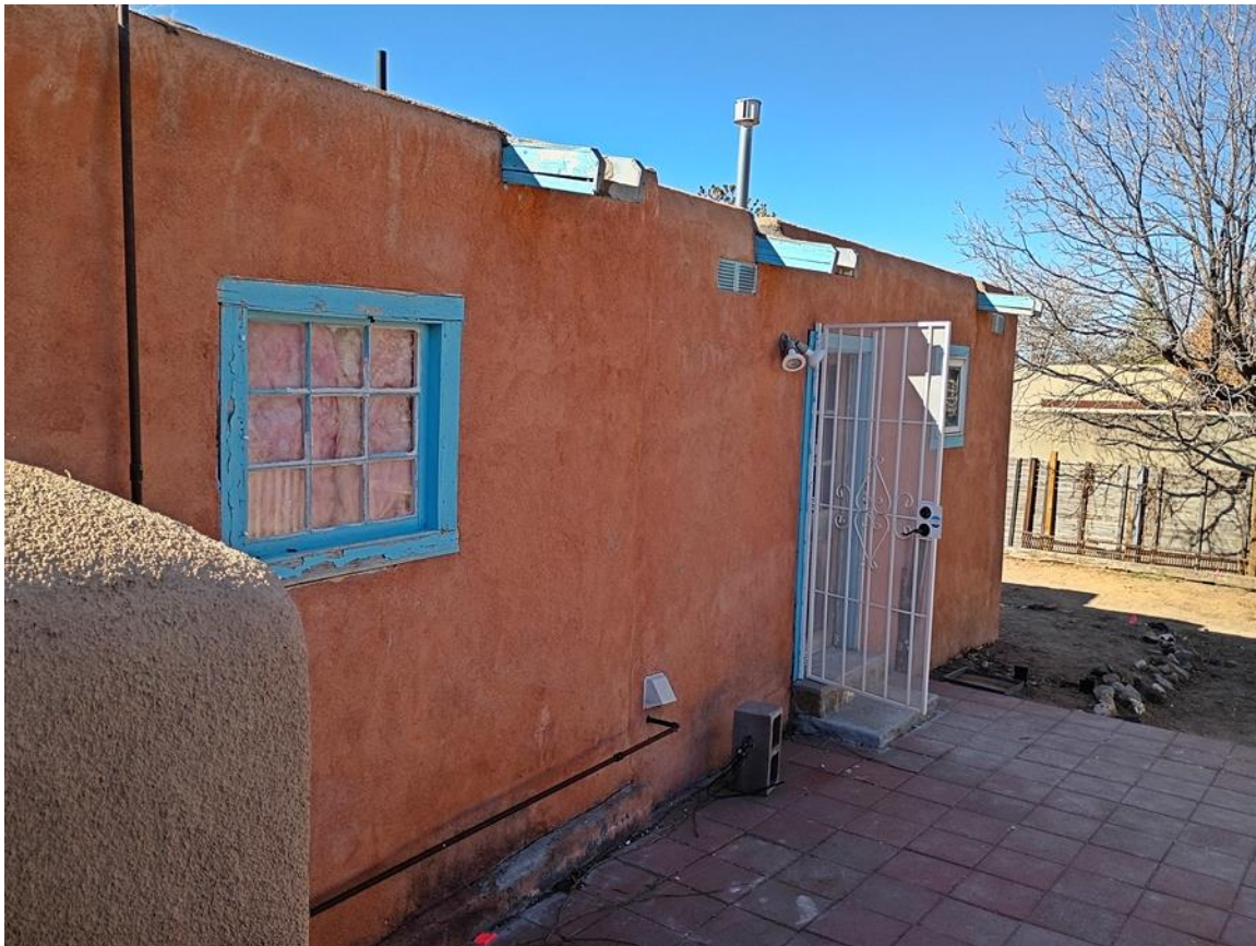
Photo 6: North elevation, Camera facing southwest.
