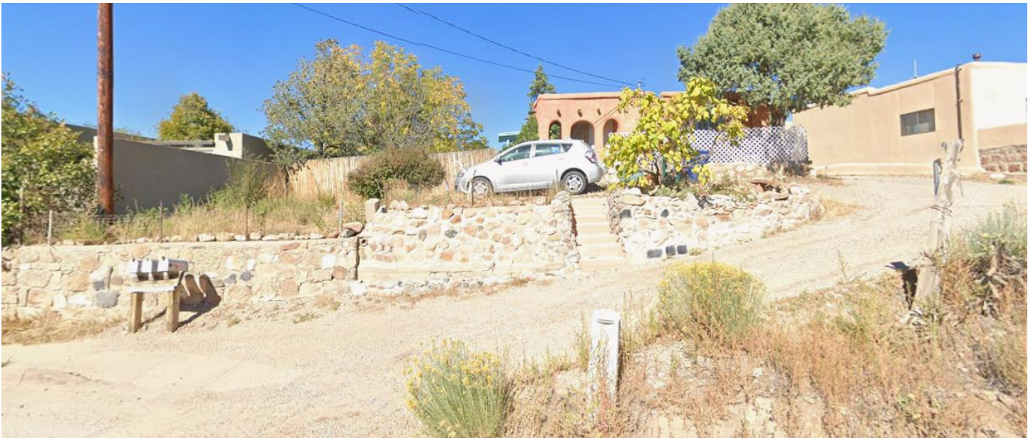
Figure 2: Street View of Property showing the retaining walls
