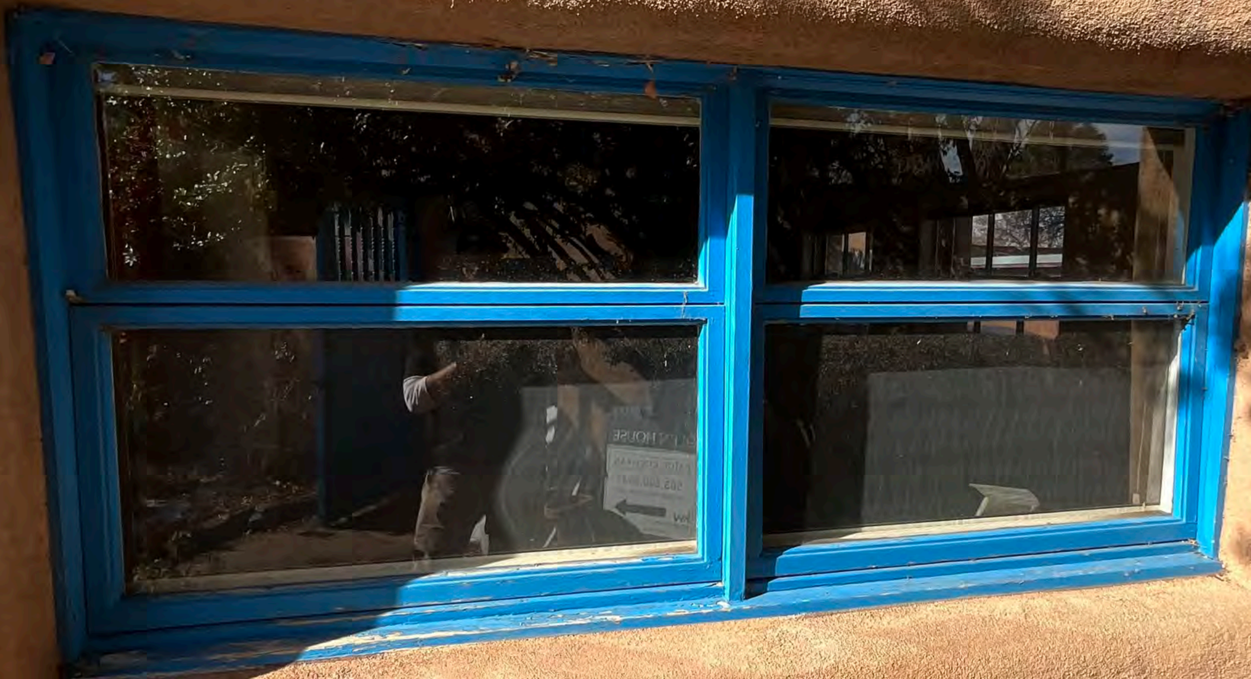
East Elevation Window W14
