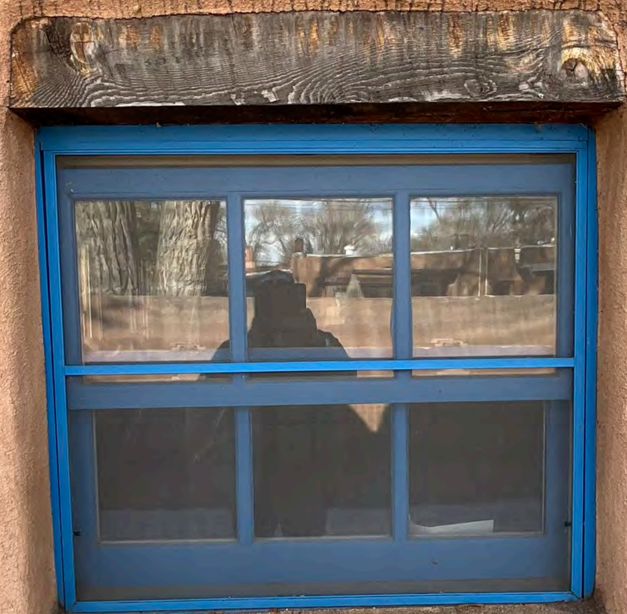
North Elevation Window W12
