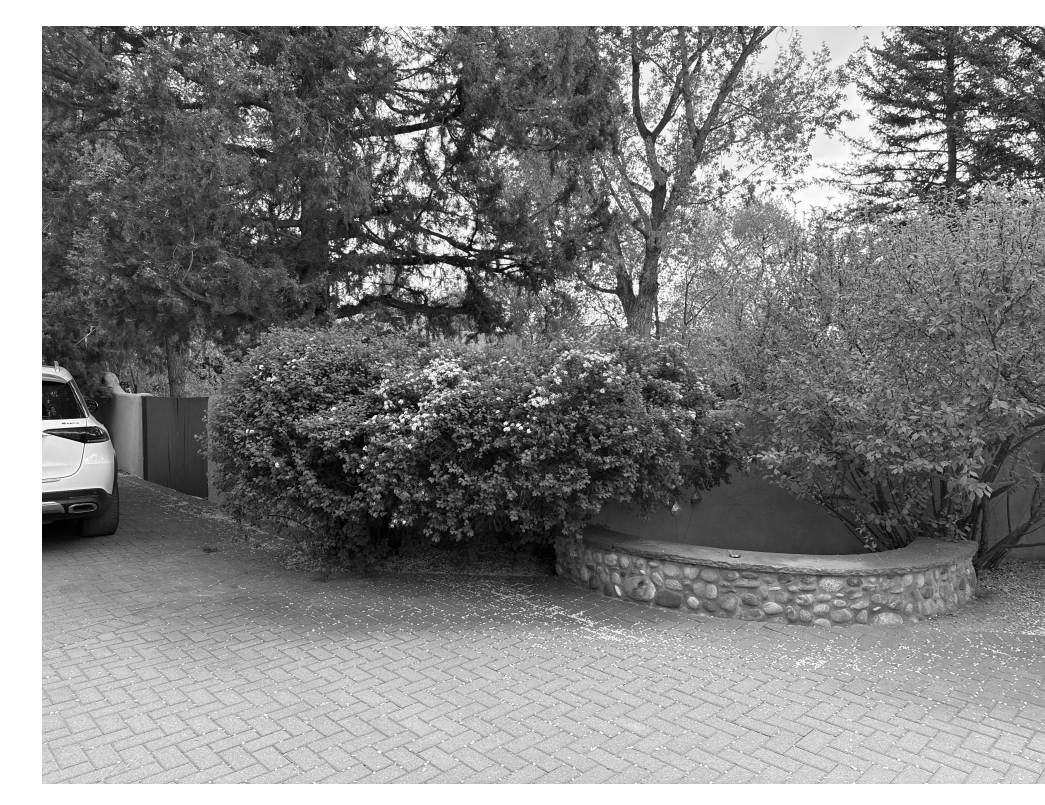
PORTION OF WALL AT NEW OPENING
