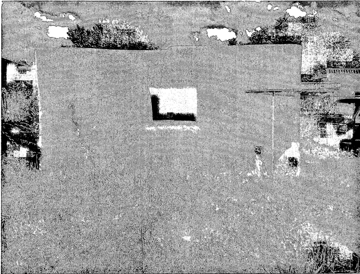
Figure 6: West elevation, facing east. September 16, 2015.
