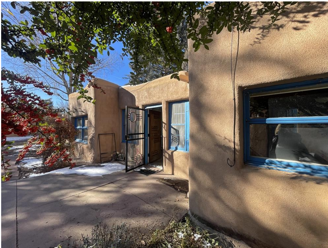
Photo 5: East elevation. Camera facing southwest.
