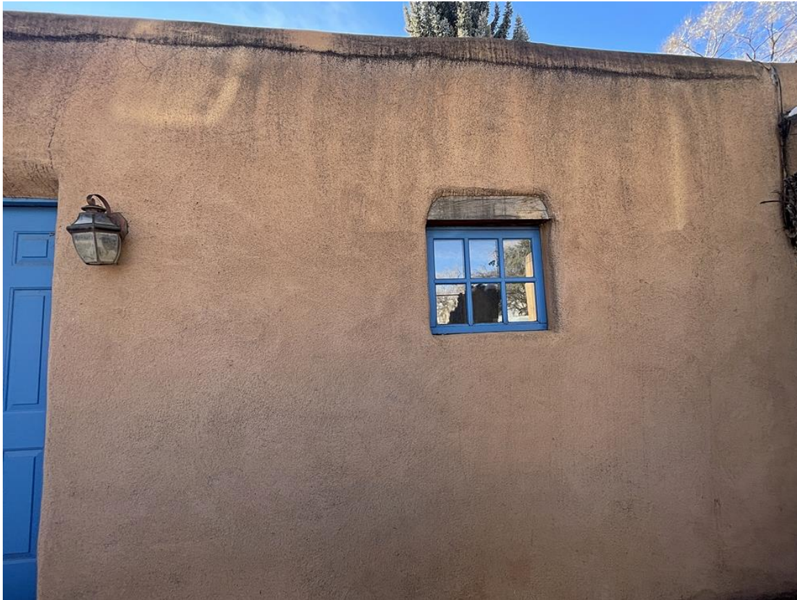
Photo 15: North elevation. Change of fenestration after 1992. Camera facing south.
