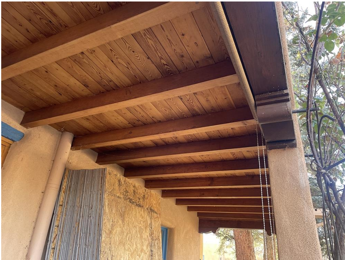
Photo 12: West elevation. Portal decking. Camera facing up.
