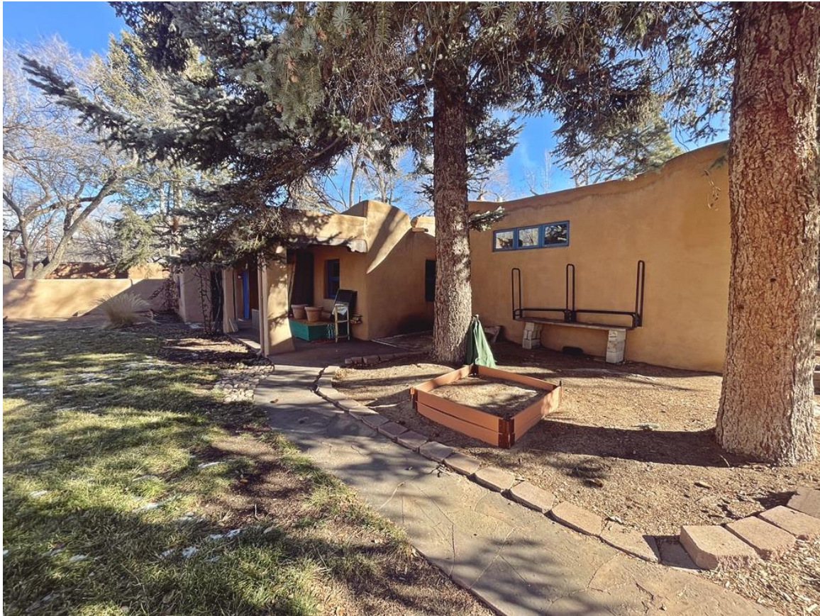
Photo 9: West elevation. 1992-93 addition at right. Camera facing northeast.
