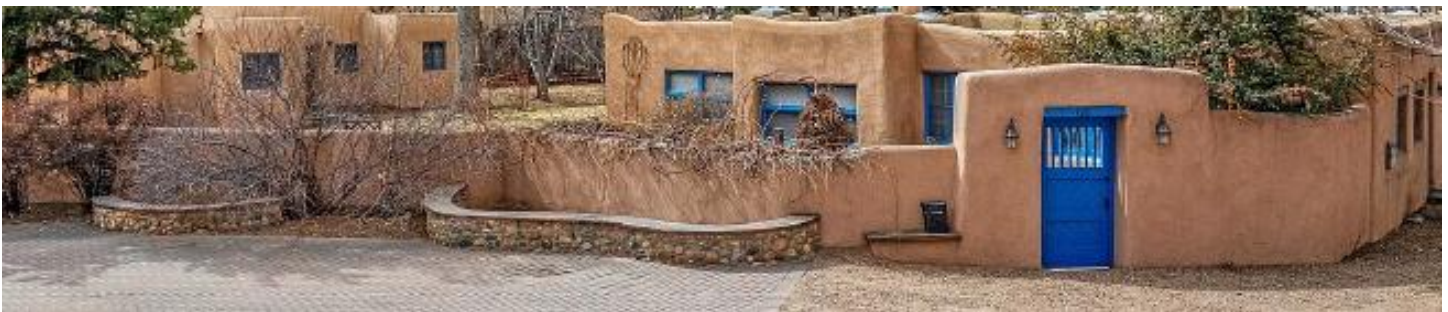
Figure 3: East Yard wall: planter on left is approximate location of proposed opening
