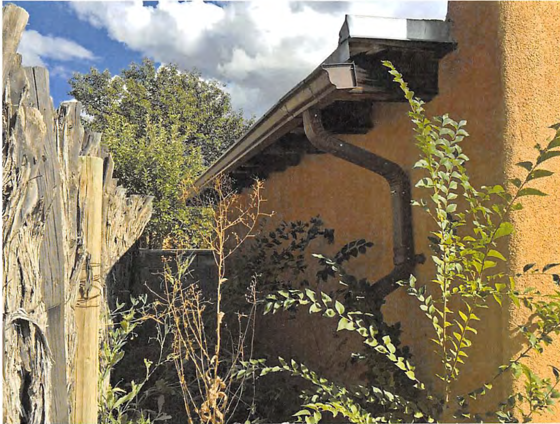
Figure 10: North elevation, facing east. October 6, 2016.
