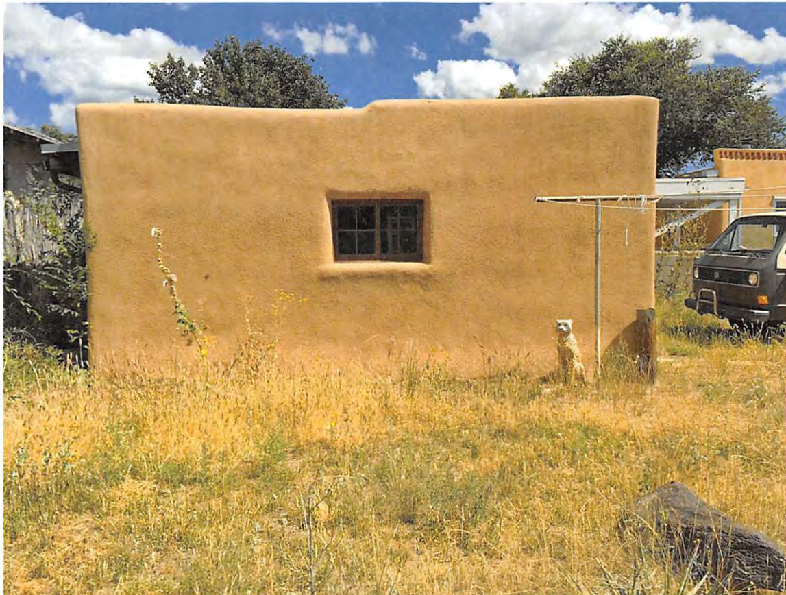
Figure 6: West elevation, facing east. September 16, 2015.
