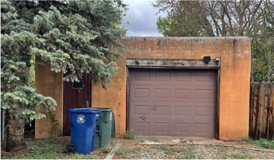
Figure 3: South Elevation of Accessory Structure
