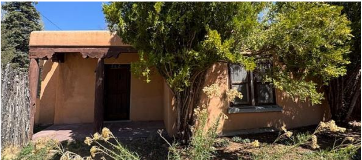
Figure 2: South Elevation of Residential Structure
