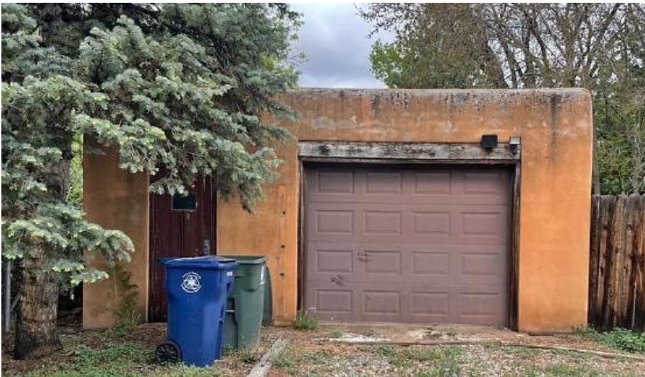
Figure 3: South Elevation of Accessory Structure
