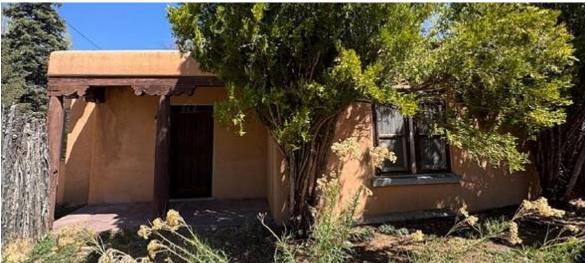
Figure 2: South Elevation of Residential Structure
