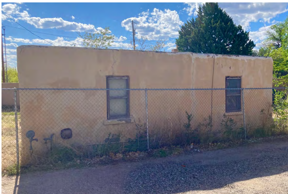
East façade – looking west – May 2025
