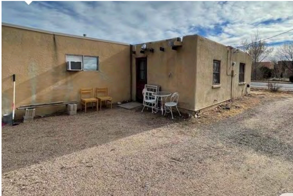
Wood framed addition – pre collapse - 2023
