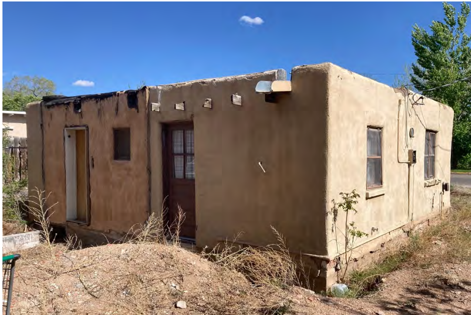
Northwest corner – looking southeast – May 2025
