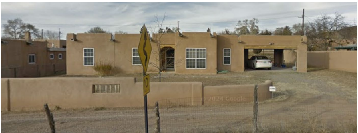
Figure 2: Street view 1226A Cerro Gordo Road
