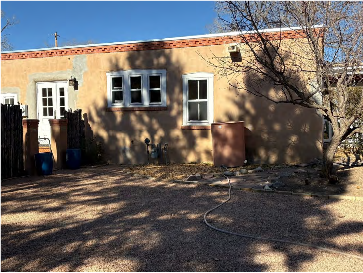
View Facing North toward Main house
