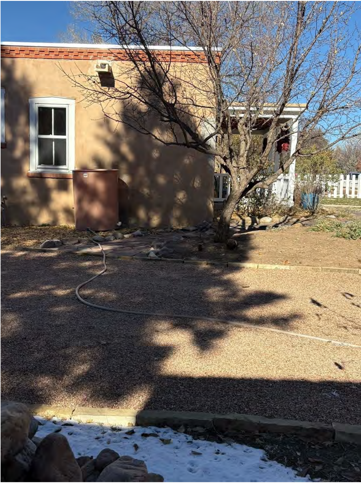
View Facing North toward Main house
