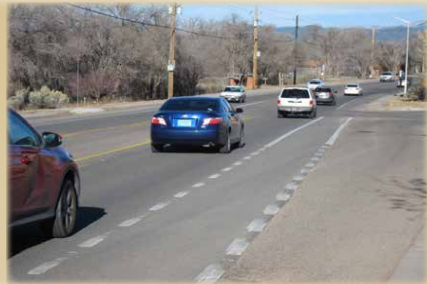
Agua Fria Street: Looking east at La Cieneguita; 3-lanes with Bike Lane / Shoulder
