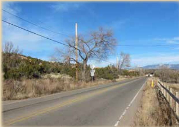
West Alameda Street: Rural Section, looking east at Nelson Loop 2 lanes, no shoulder.
