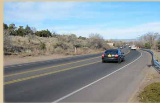
West Alameda Street: Semi-Rural Section, looking east at Calle Nopal; Striped Median w/ Shoulder, Sidewalk and Streetlights only on south side of roadway.
