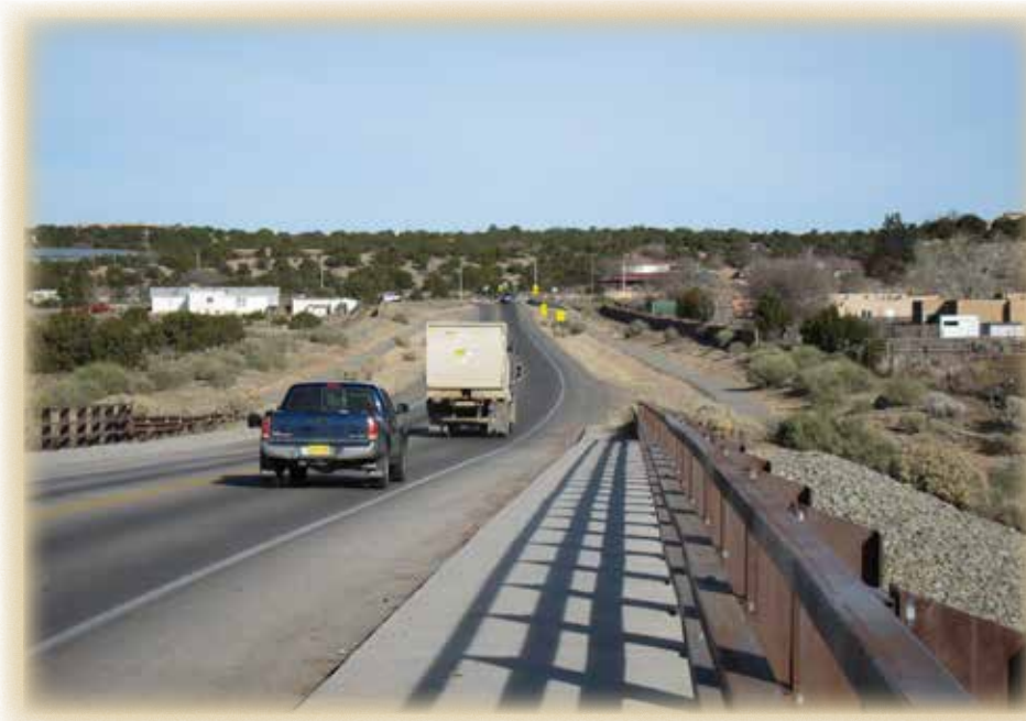
Siler Road: Looking north toward West Alameda; 2-lanes, paved shoulders, multi-use trails.
