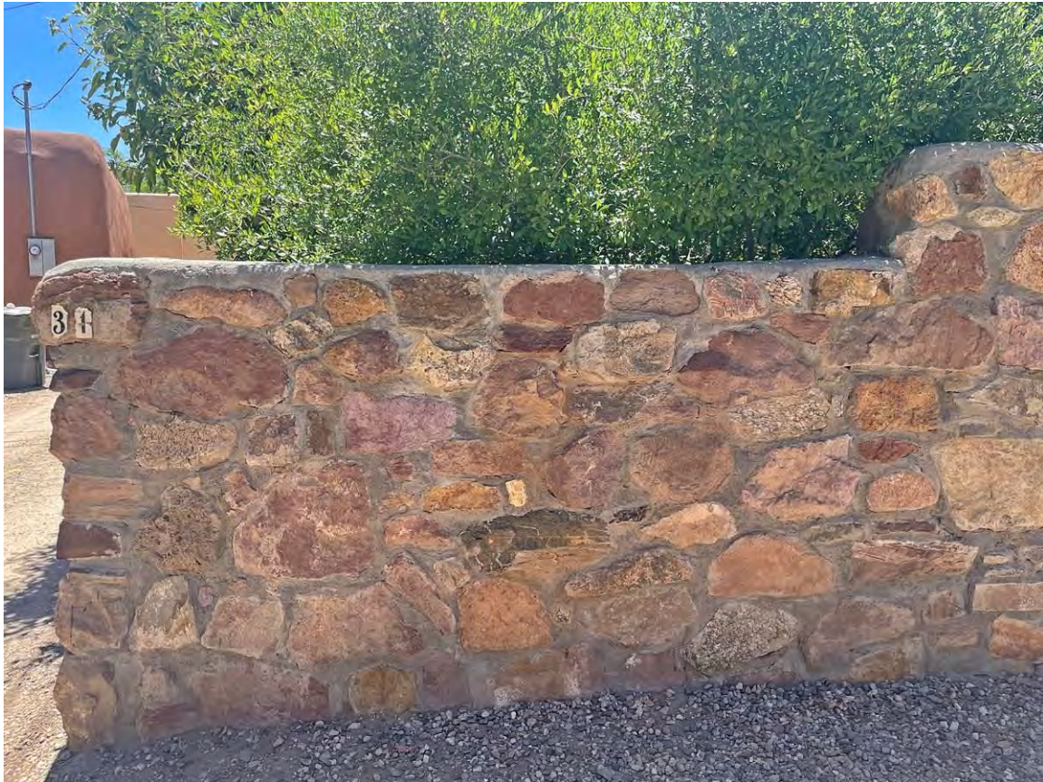
Photo 15: Recently constructed stone wall section, west elevation. Camera facing east.
