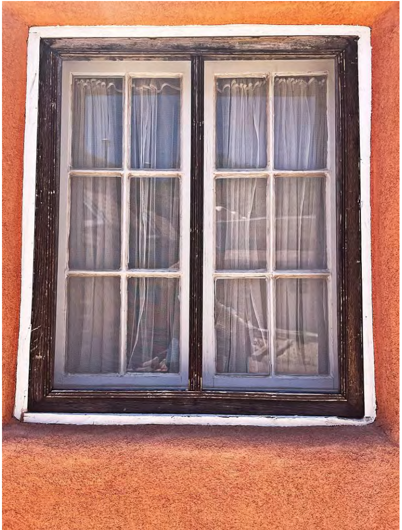
Photo 5: North elevation, casement windows. Camera facing south.
