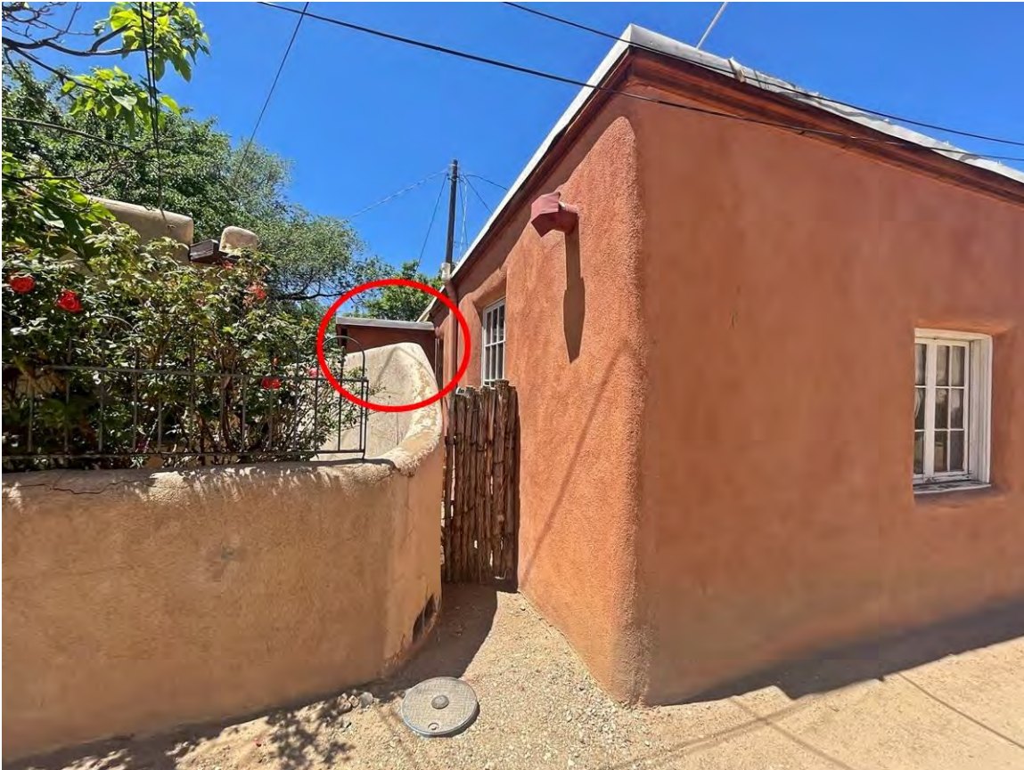
Photo 13: East elevation oblique. Camera facing southwest. 1970s closet addition highlighted. Note single sash casement at center.
