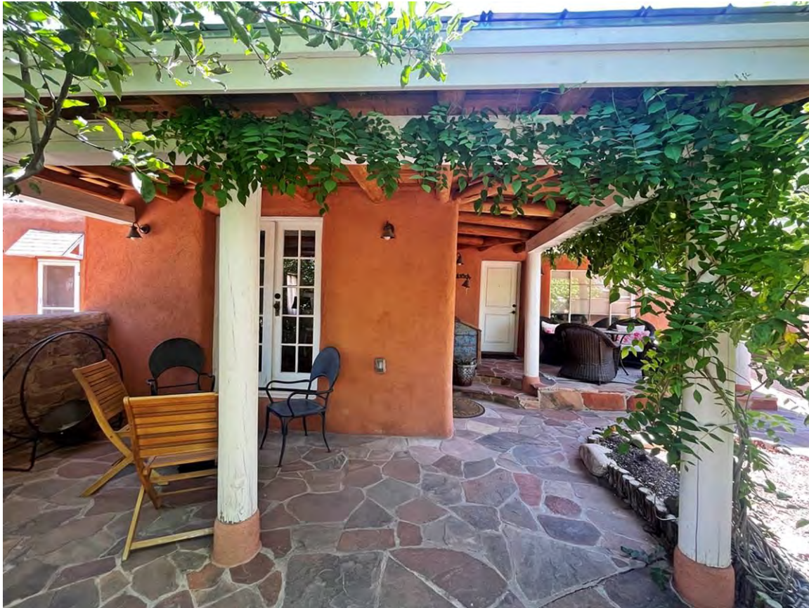
Photo 6: West elevation, northwest corner. Camera facing east.
