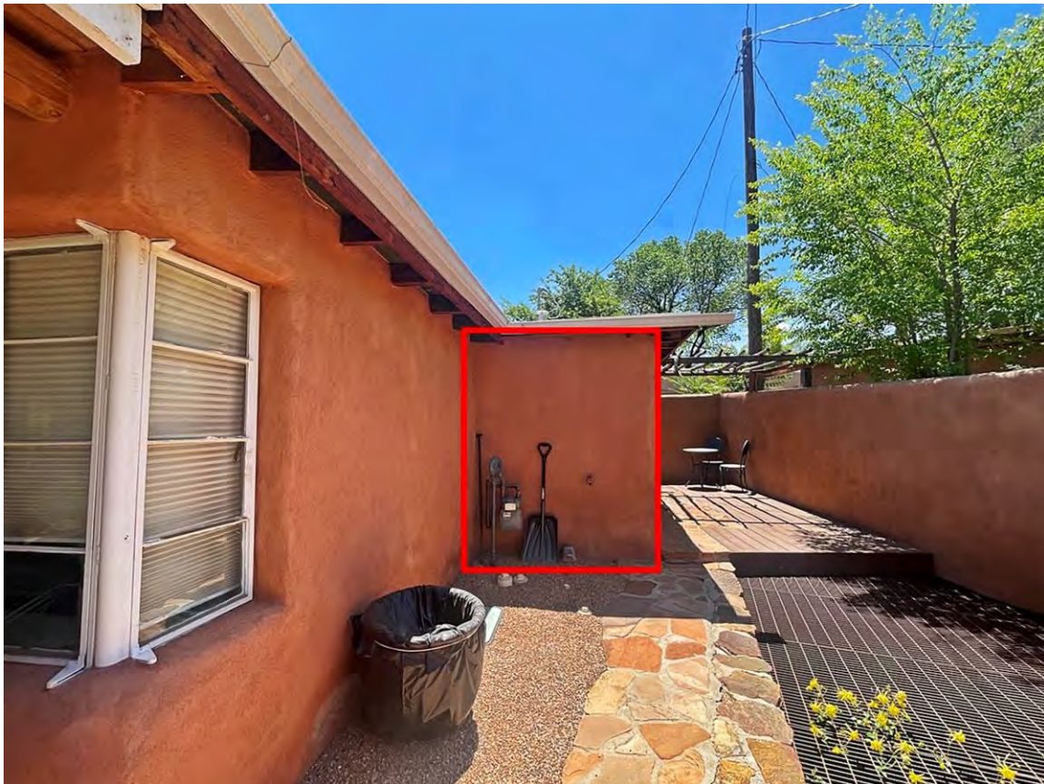
Photo 9: South elevation oblique. 1970s bump-out highlighted. Camera facing east.
