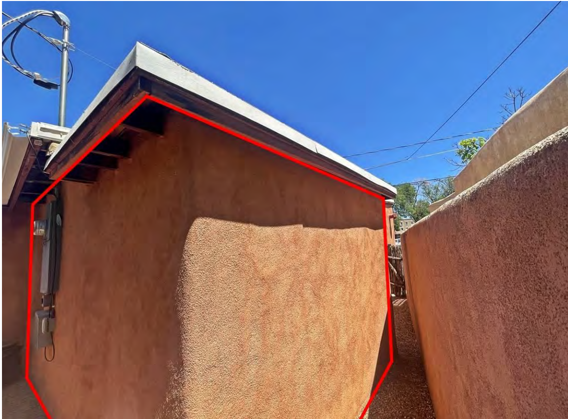
Photo 14: East elevation. 1970s closet addition highlighted. Camera facing northwest.
