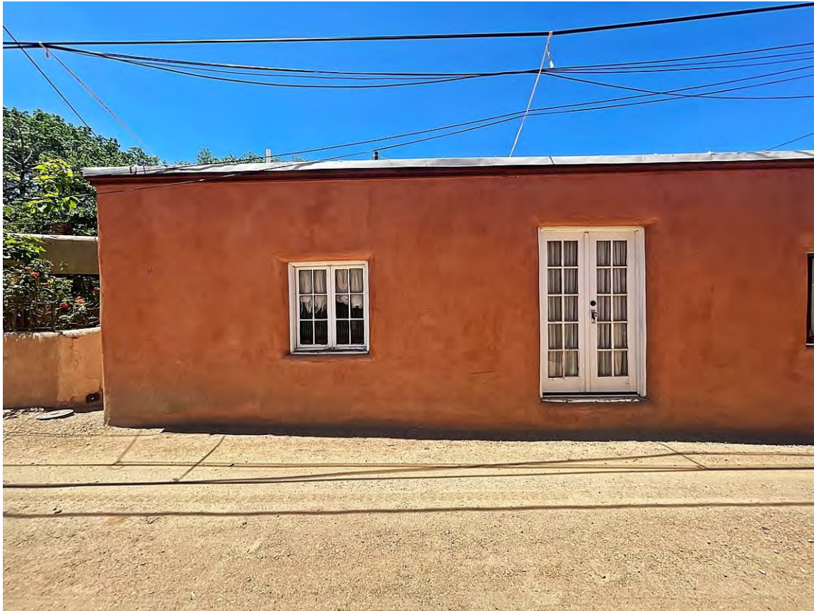
Photo 4: North elevation, east section. Camera facing south.
