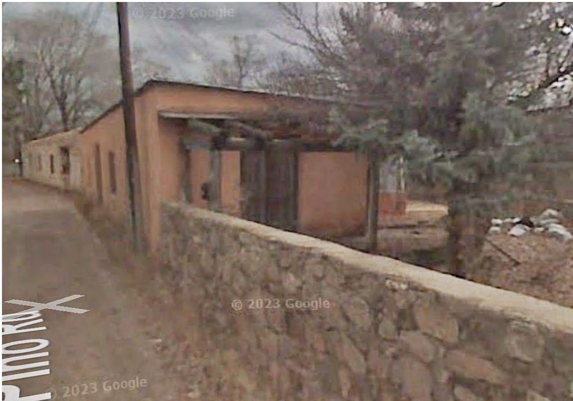
Figure 12: December 2007 Google Street View image of northwest porch.
