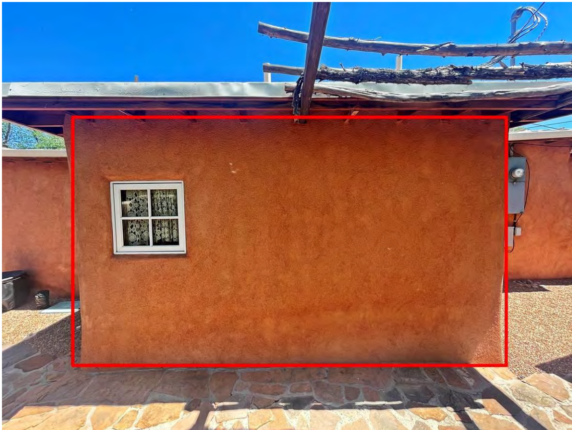
Photo 11: South elevation, middle section. 1970s bump-out highlighted. Camera facing north.
