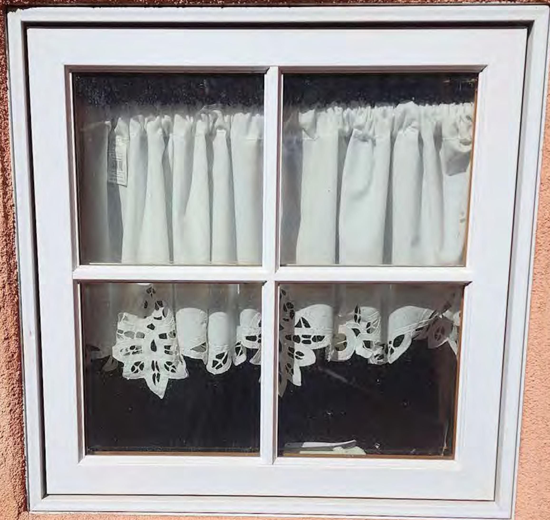
East Elevation Window C
