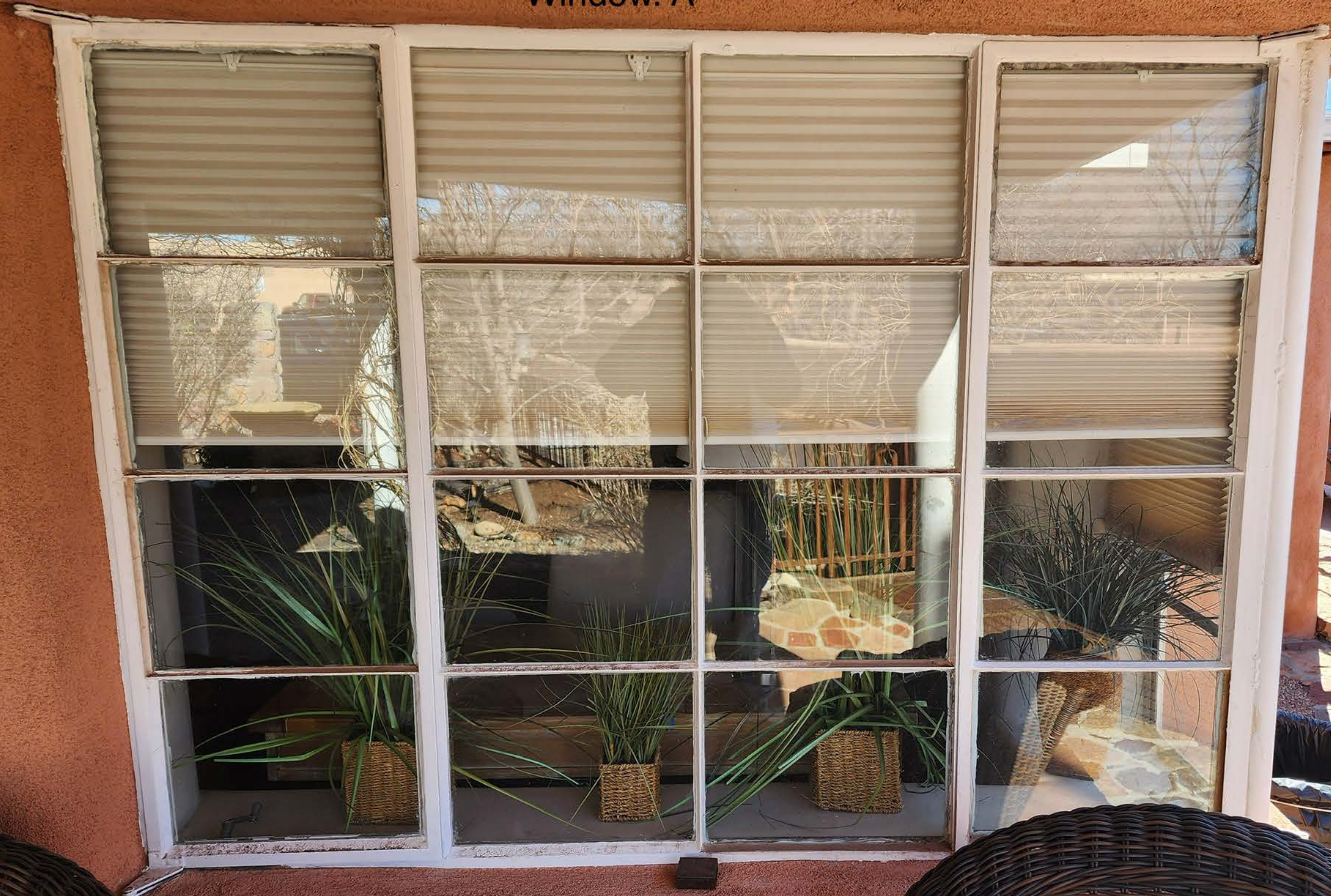
South-West Elevation Window. A
