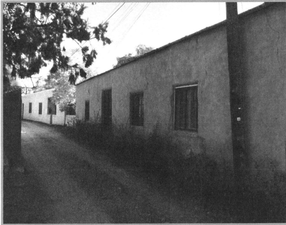
This is a continuation of the North elevation, along Pino Road.
